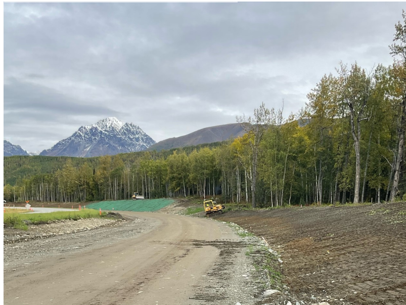
Above: Slope restoration
