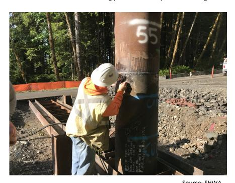
The spliced sections of pile are welded together and are inspected with an ultrasonic testing instrument to verify there are no defects in the weld
