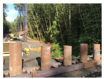
Pictured above are the first sections of the pile after being driven into the ground at abutment 2 at the Canyon Creek site.
