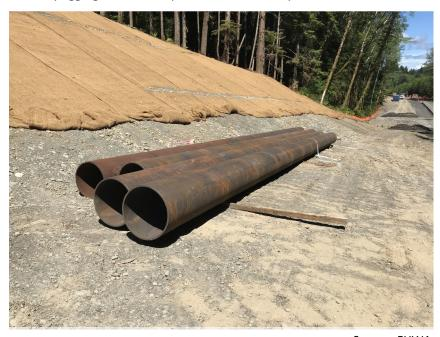
Source: FHWA Pictured above are a portion of the pipe piles that were delivered this week in preparation for pile driving next week.
