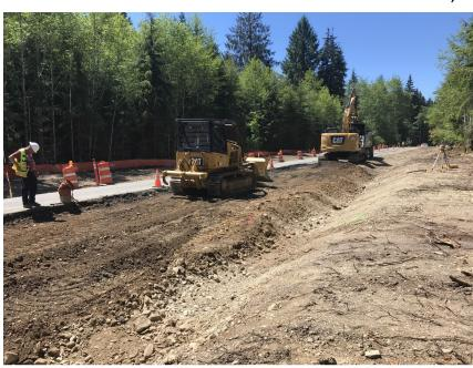
Source: FHWA East side of Canyon Creek site after the asphalt was removed and before the roadway aggregate base was placed. This will be repaved in late summer
