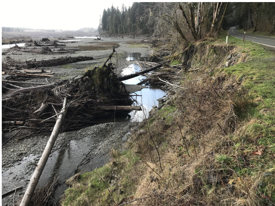
An example of a location along Upper Hoh River Road where the Engineered Log Jams will be installed to prevent bank erosion.
