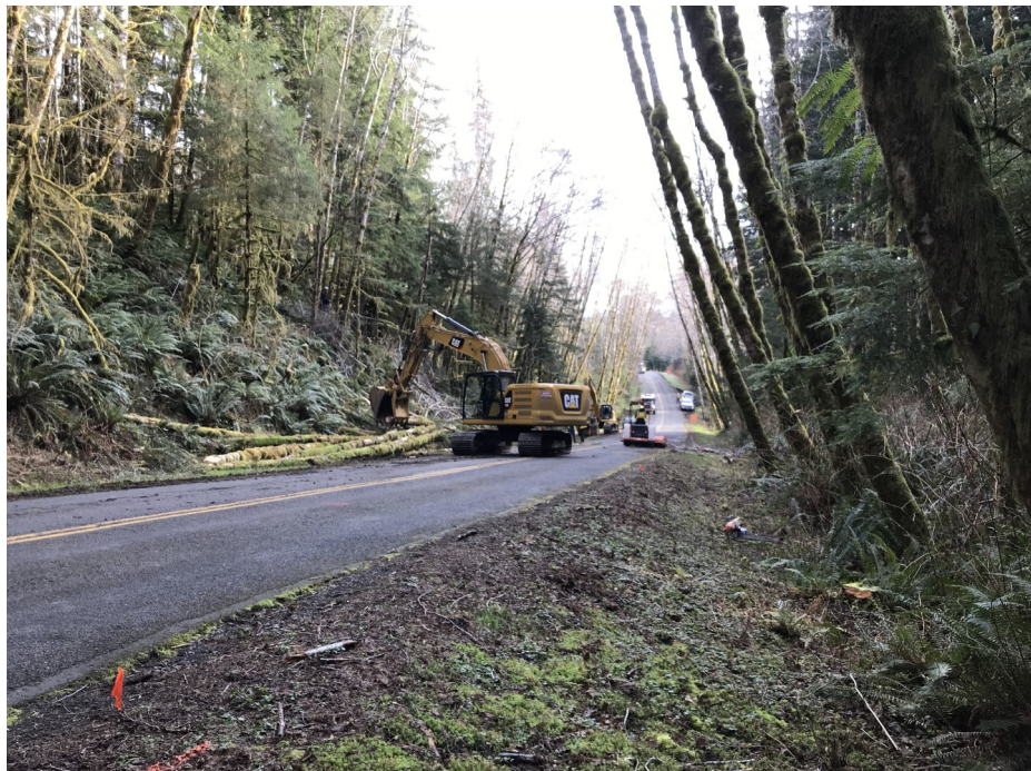
Clearing of trees at Canyon Creek for new bridge construction
