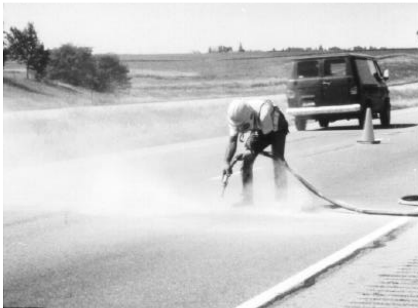
Figure 11. Sandblasting operation.
