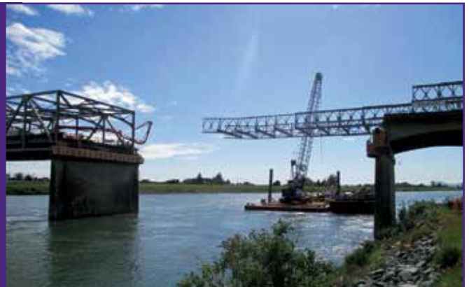
The temporary spans are shown here during installation.
