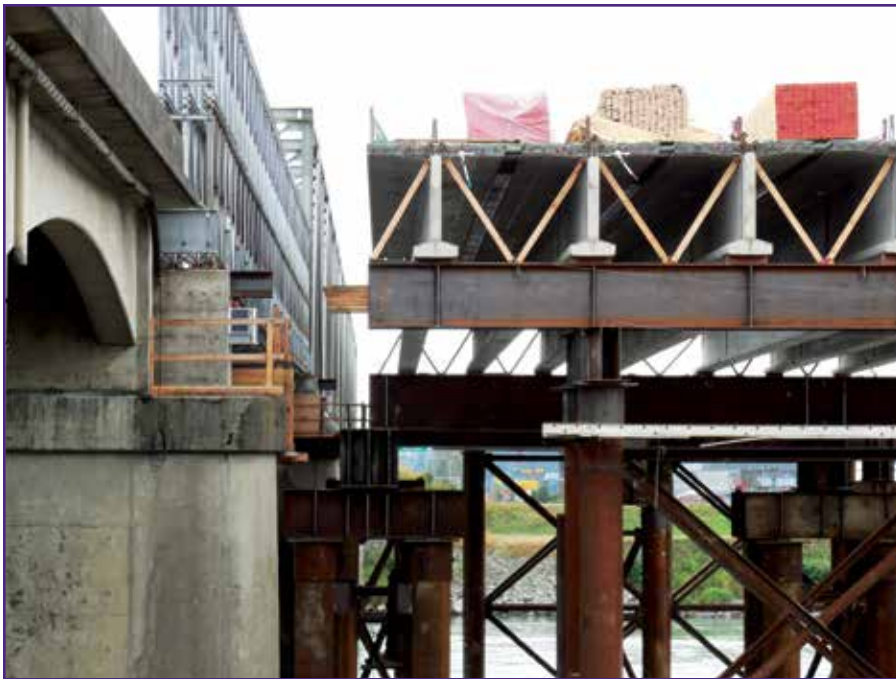
The design-build team constructed the permanent replacement span on a work platform (right) next to the temporary side-by-side spans (left).
