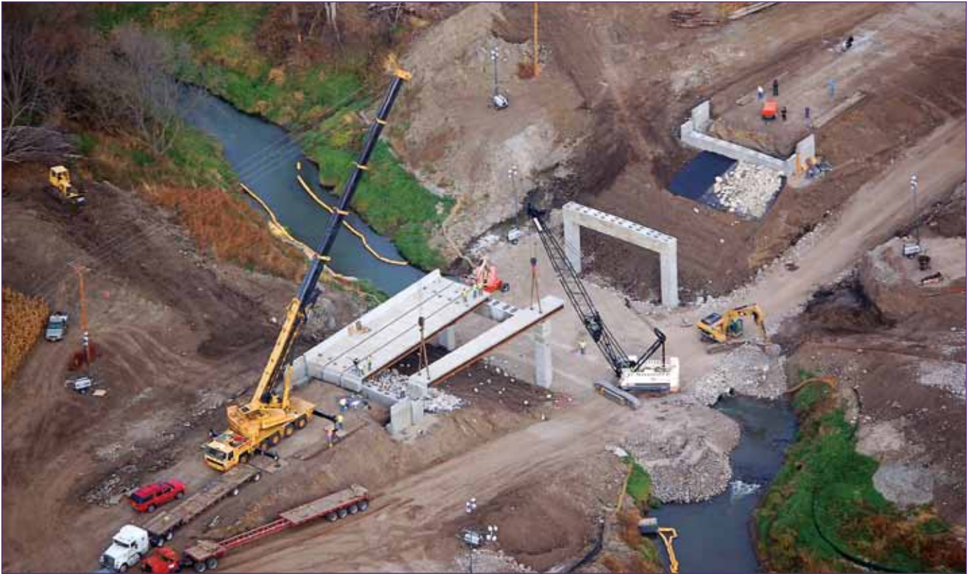
This crane is lowering a concrete bridge section onto pylons set in Keg Creek, located in western Iowa. The project is a pilot of Innovative Bridge Designs for Rapid Renewal (R04), a SHRP2 Solution for accelerating bridge construction.
