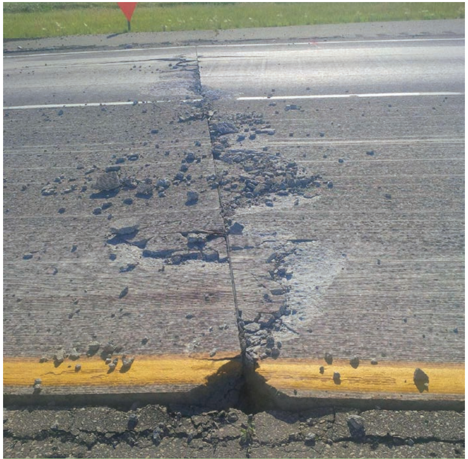
The photograph is an example of a concrete blowup near the joint of a rigid pavement. Pieces of the concrete are missing along the joint. Photo: Archie Miller, Manitoba Infrastructure.
