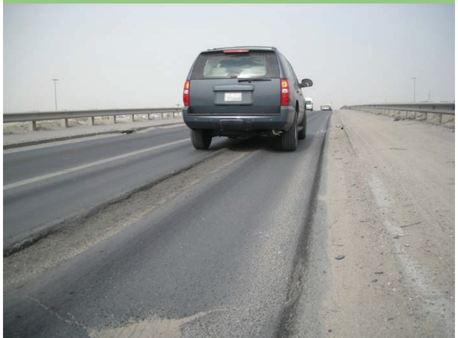
Here, a vehicle travels on a flexible pavement that has severe rutting in the asphalt pavement. The pavement is located in a desert climate outside of the United States, but clearly demonstrates deformation.
