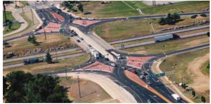
When the Missouri Department of Transportation redesigned the I-44/Kansas Expressway interchange, as shown here, it extended the medians to reduce the potential for drivers to enter going the wrong way.
