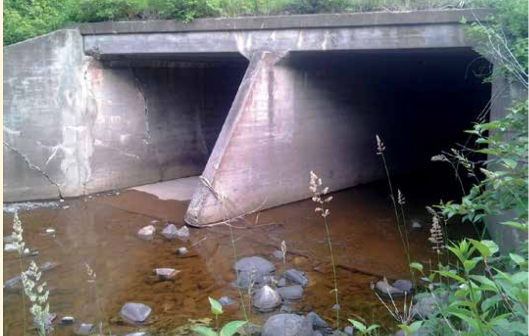
For culvert 5648, shown here, which carries MN-61 over Silver Creek in Minnesota's Arrowhead Region, the State used input from climate models indicating that a slightly larger replacement structure would be more cost effective in the long term. Photo: MnDOT.
