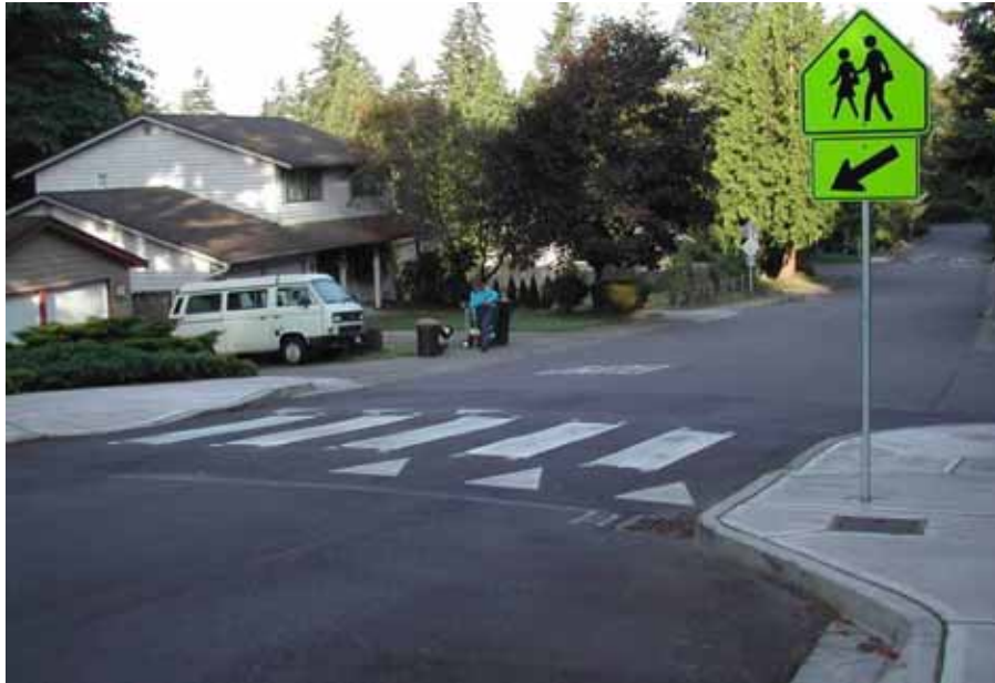
Figure 20-5. Photo. Speed humps can be combined with curb extensions and a winding street alignment.
