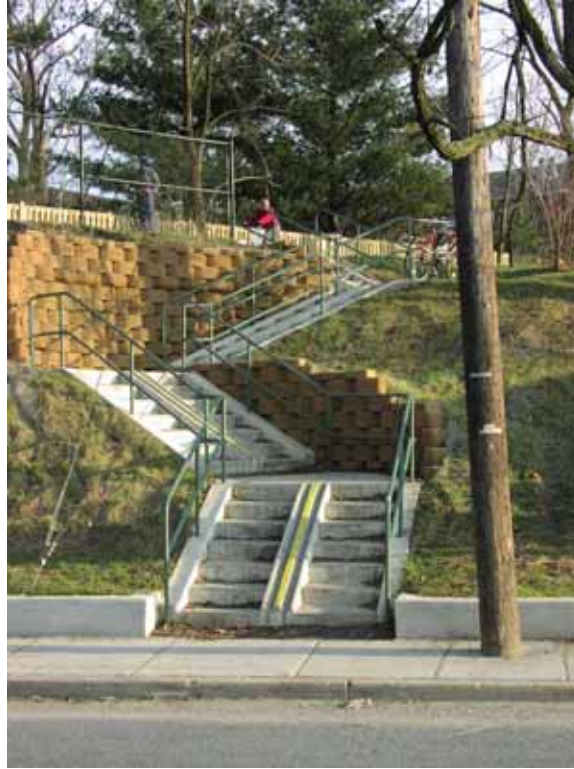
Figure 19-6. Photo. Stairway with bicycle rolling troughs (Capital Crescent Trail, Bethesda, MD).
