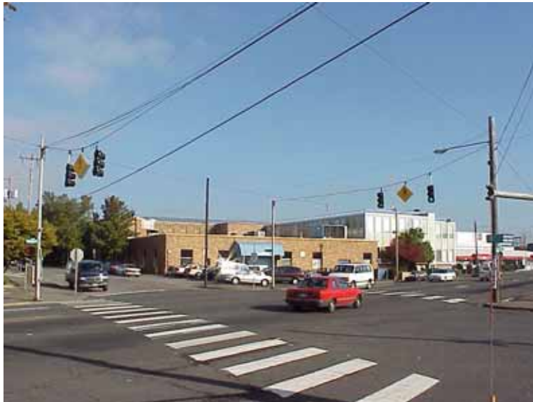
Figure 11-9. Photo. Half-signal in Portland, OR.
