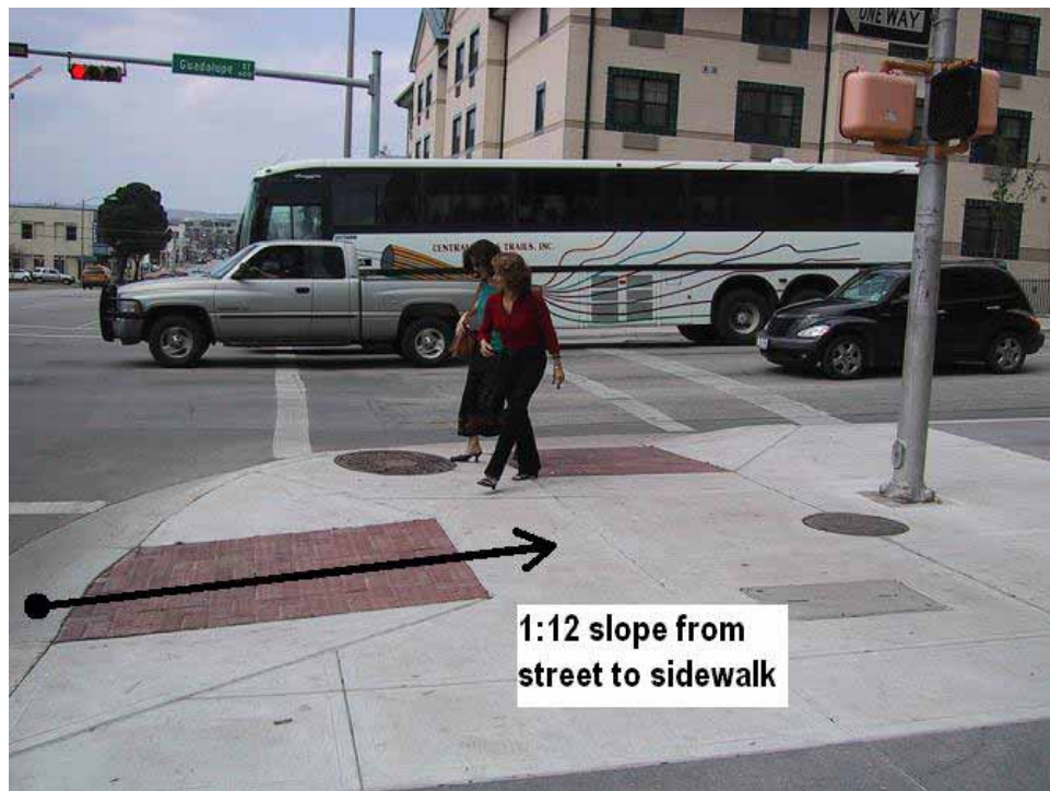
Figure 8-15. Photo. Perpendicular curb ramp.
