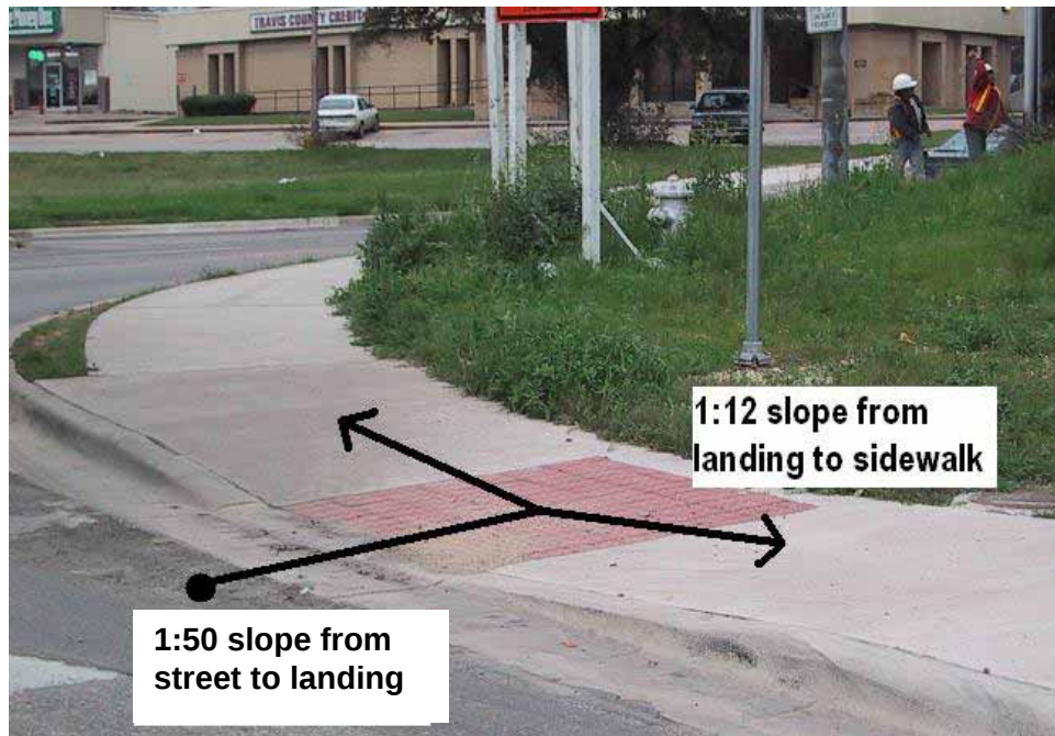
Figure 8-16. Photo. Parallel curb ramp.
