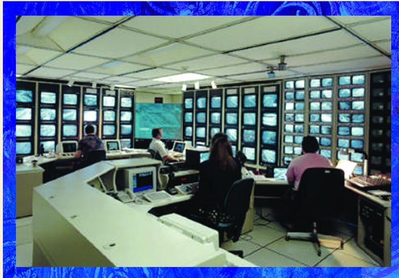
*Traffic management centers, like this one, use data from road sensors, cameras, and other sources to adjust traffic flow.*
