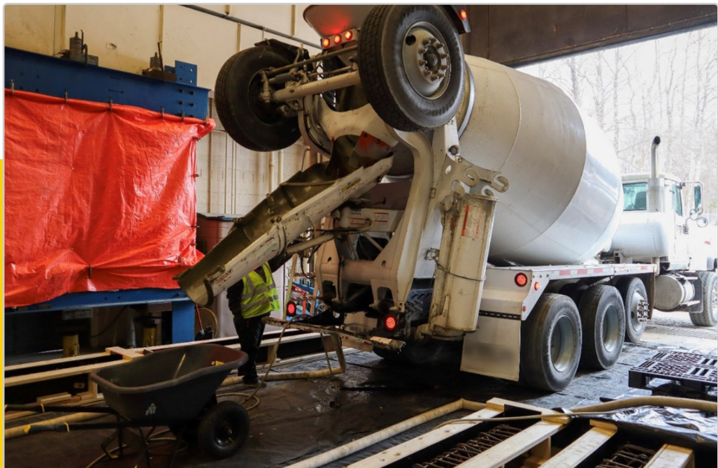
Source: FHWA. The industrial ready-mixed concrete truck charged with the first batch of LC2 concrete.
