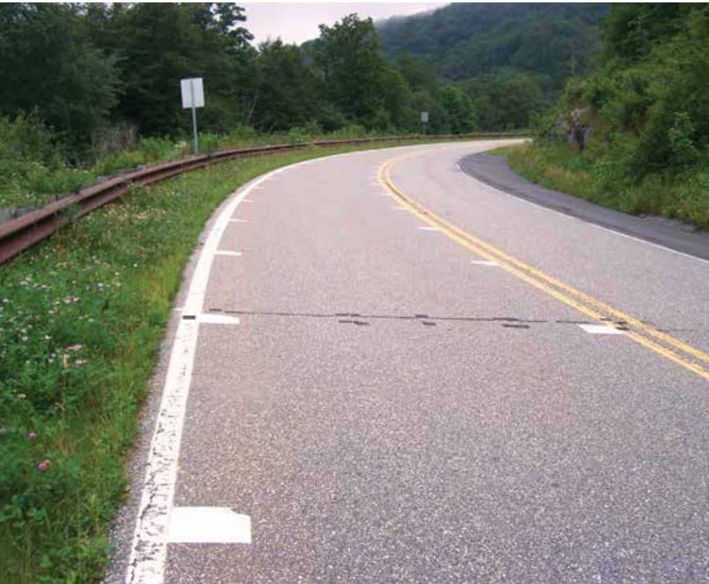
Speed-reduction pavement markings installed by the North Carolina Department of Transportation (NCDOT) give road users the illusion that they are going faster than they are to encourage motorcyclists to slow down as they traverse tight curves. The wide apron installed on the inside of the curve serves to collect gravel that washes down from the hillside, keeping this hazard off the roadway. *Photo: NCDOT.*
