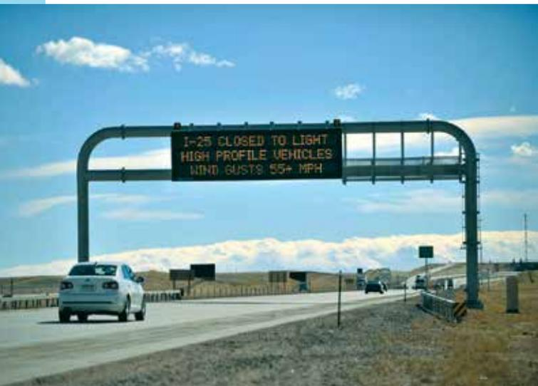
**This dynamic message sign displays a wind warning and vehicle restriction to drivers in Wyoming.**
