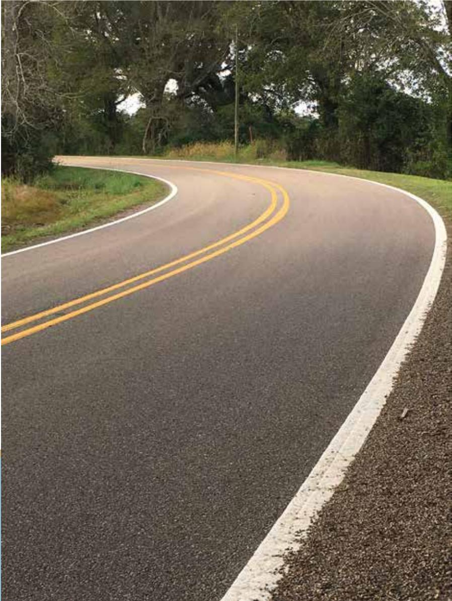
Carefully maintaining the brightness and retroreflectivity of a 6-inch (15-centimeter) white edge line like the one shown along this roadway can provide positive guidance to help motorists navigate tight horizontal curves more safely.
