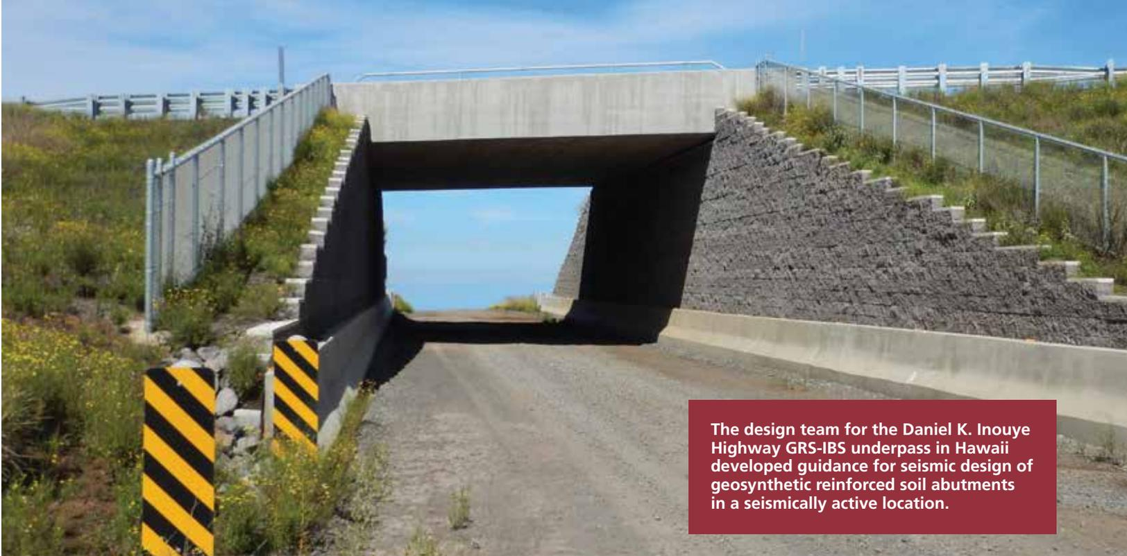
The design team for the Daniel K. Inouye Highway GRS-IBS underpass in Hawaii developed guidance for seismic design of geosynthetic reinforced soil abutments in a seismically active location.
