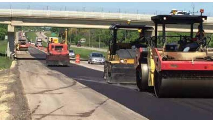
The Minnesota Department of Transportation used roller compactors, shown here, equipped with intelligent compaction instrumentation to monitor the densification of its test sections. Photo: MnDOT.
