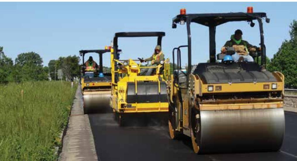
**The Pennsylvania Department of Transportation employed these three vibratory steel wheel roller compactors operating in an echelon formation to help achieve increased density targets for its demonstration test sections.**
