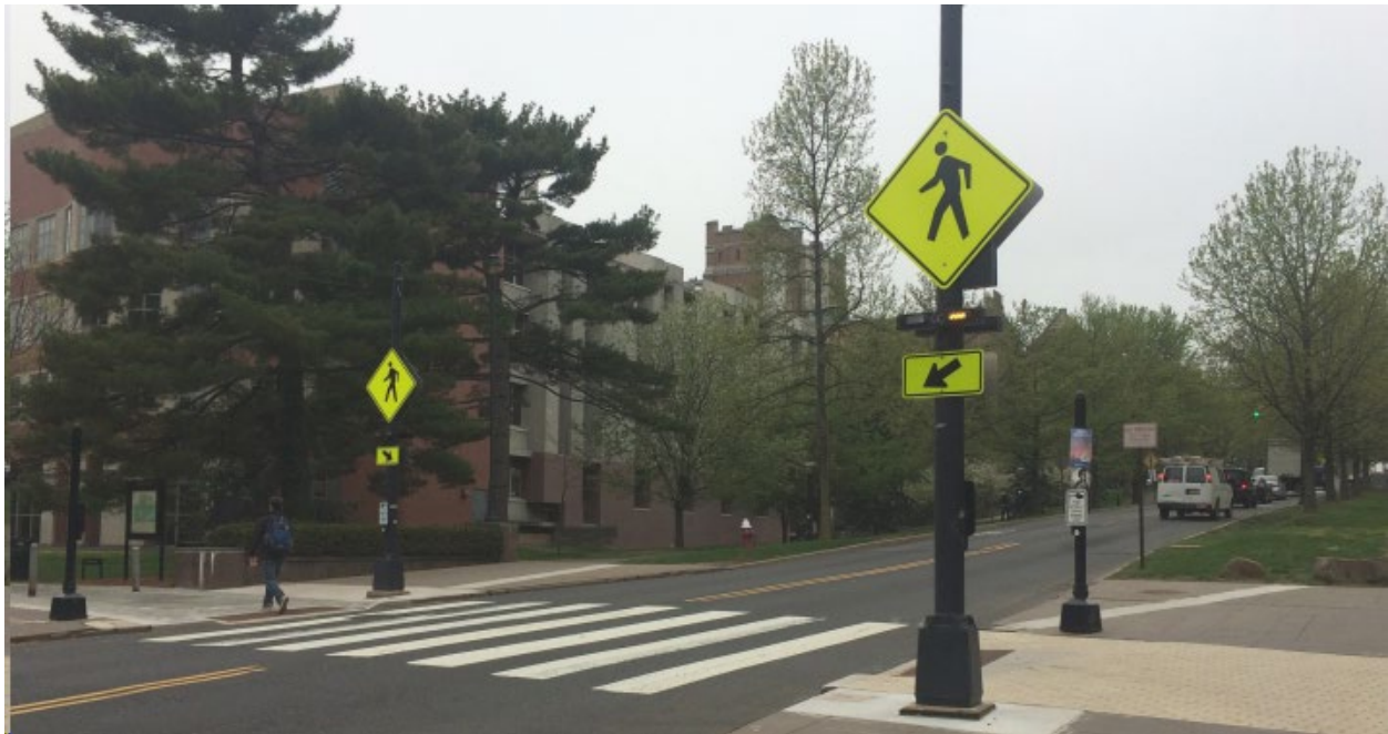
Figure 30. Photograph. Rectangular Rapid Flashing Beacon (RRFB). Source: FHWA.
