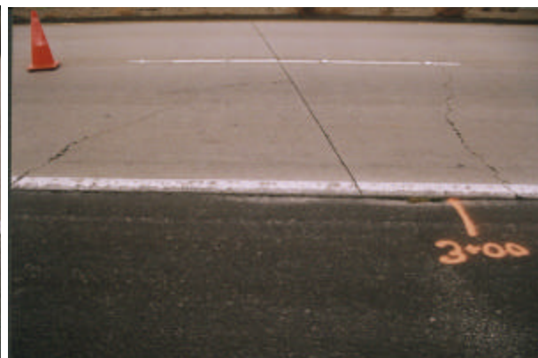
Figure 3.1.11 Corner break near approach joint at 06-CS1, Tracy Test Road (control section).
