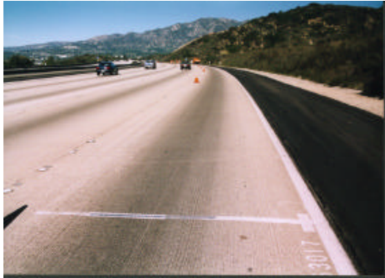
Figure 3.1.4 Overview of test site 06-3017.
