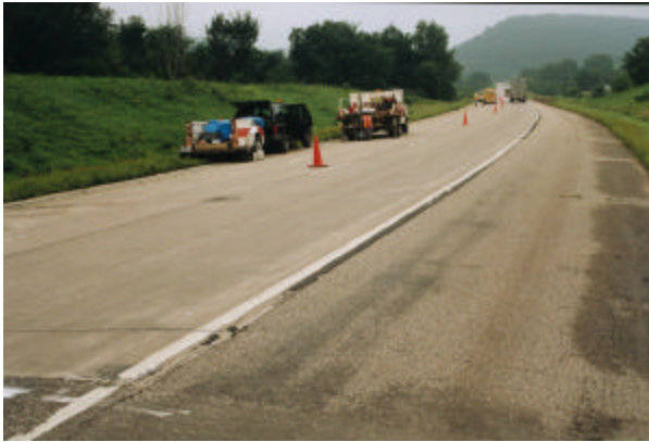
Figure 3.1.22 Overview of test site 27-4054.
