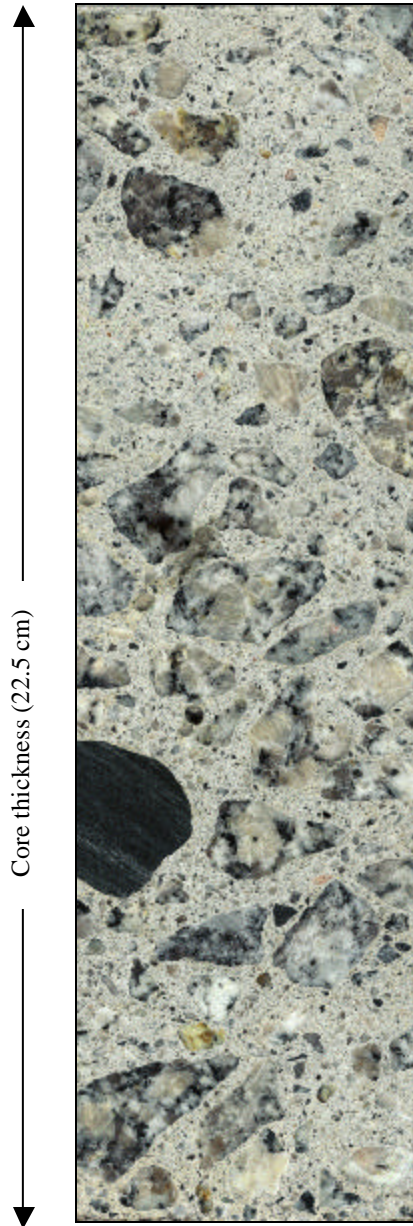
Figure 3.2.15 Polished cross-section of pavement section 13-GA1-5.
