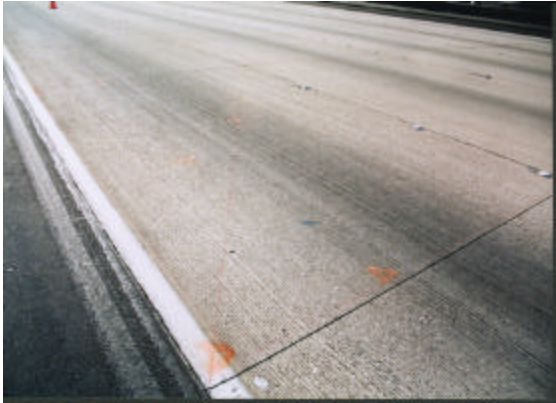
Figure 3.1.5 Distress free slab and joint in test site 06-3017.
