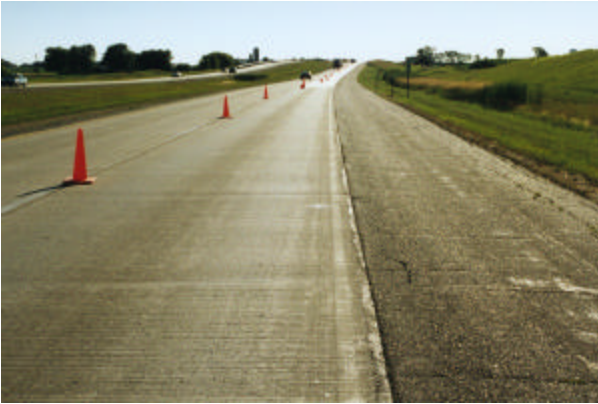
Figure 3.1.26 Overview of test site 55-3008.
