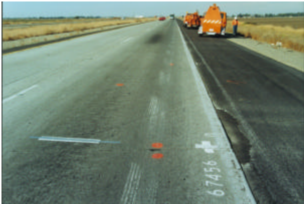
Figure 3.1.8 Overview of test site 06-7456, Tracy Test Road.
