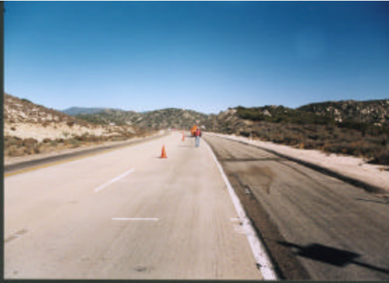
Figure 3.1.6 Overview of test site 06-3021.
