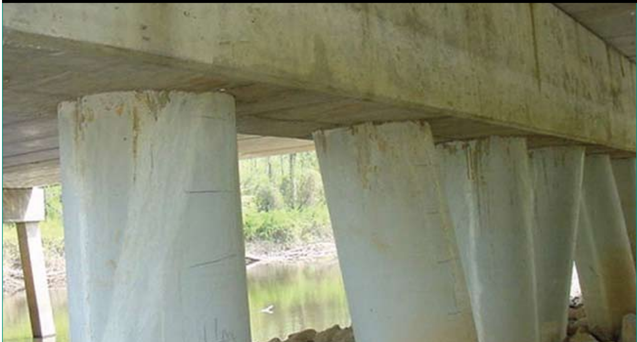
Figure 7. Fiber reinforced polymer concrete filled shells used for lightly loaded structures.
