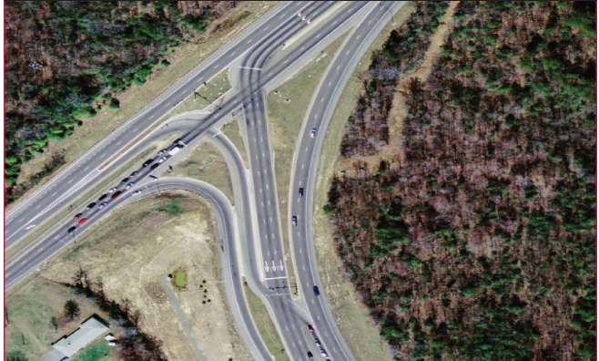
Figure 3. A 3-legged partial DLT intersection in Accokeek, MD.
