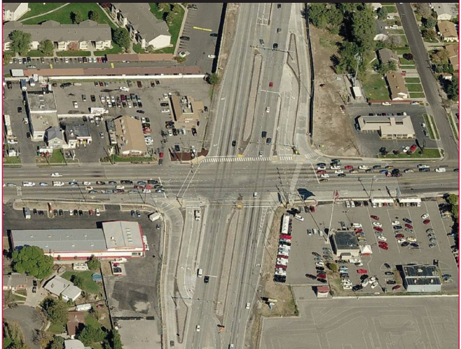
Figure 4. DLT intersection in Salt Lake City, UT.
