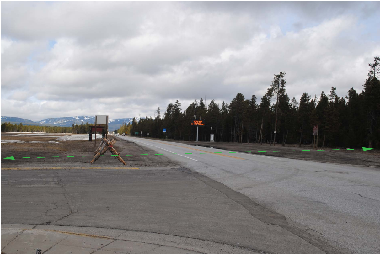
Figure 3.4. Intersection of Iris Street with US 20 (Targhee Pass Highway), looking west.
