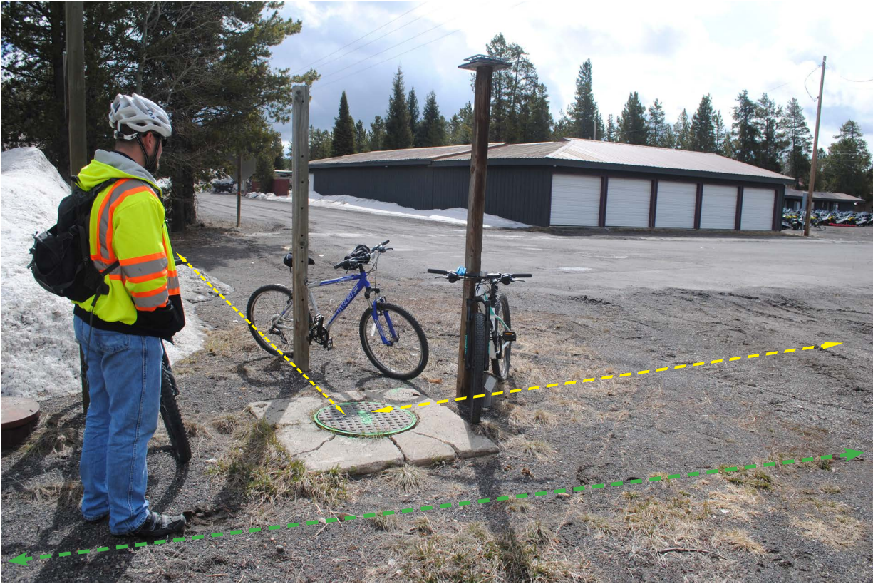
Figure 4.5. Intersection of Iris and Alley D/D Parkway, looking southeast. The utility access shown is a Town water line that aligns with the two streets as approximated by the dashed line.
