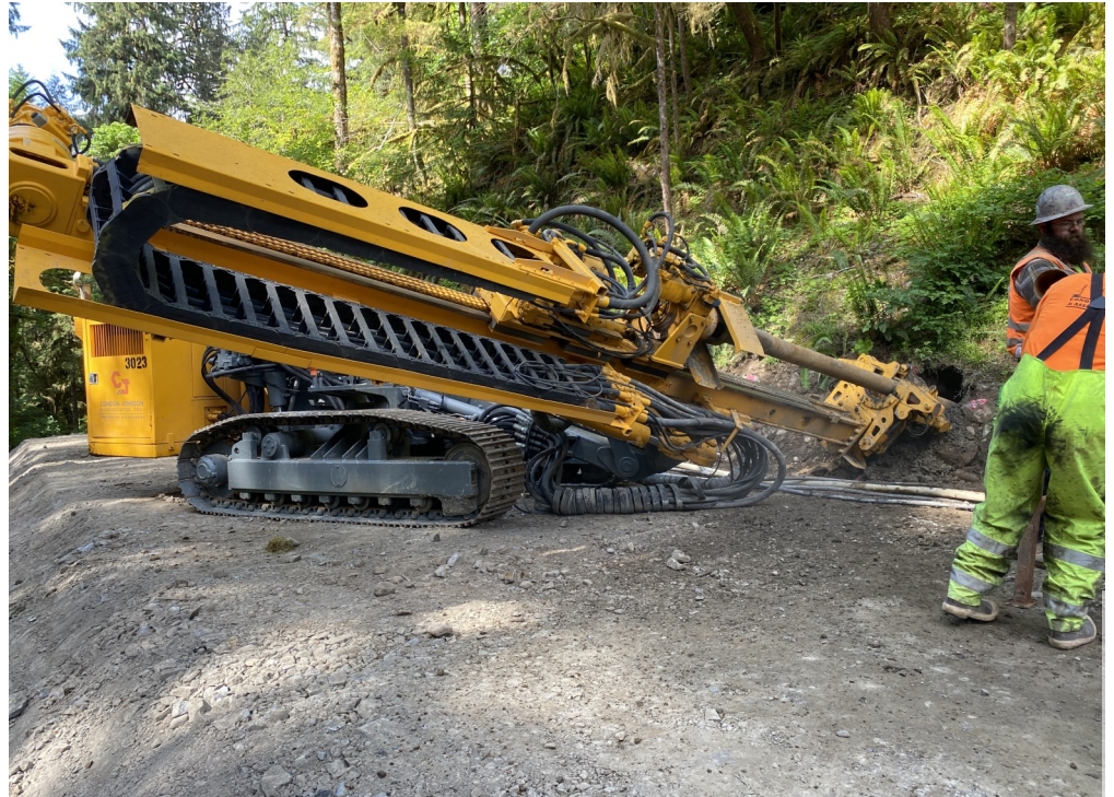
Drilling the holes for the Soil Nail Retaining Wall at the MP 7.8 site
