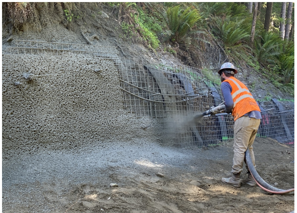
Applying the Shotcrete on the first row of Soil Nails
