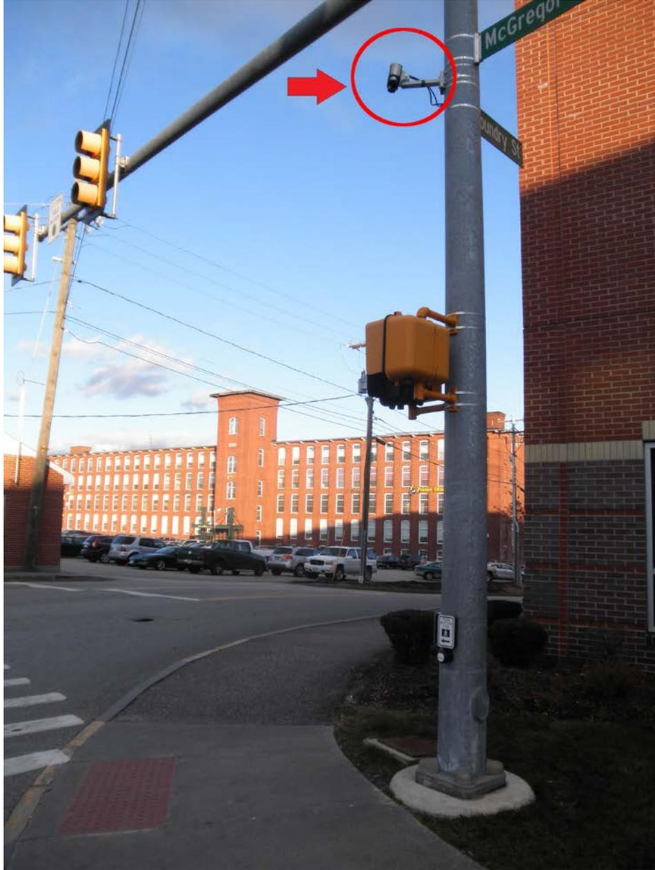
**Figure 27. Photo. Operational stereo pedestrian detection system on southeast corner of McGregor Street and Foundry Street in Manchester, NH.**
