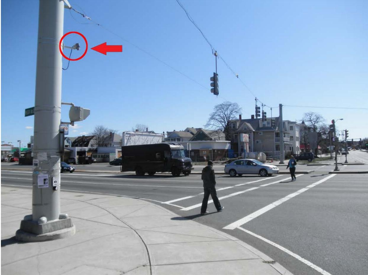
**Figure 21. Photo. Operational stereo pedestrian detection system at the north crosswalk across McGrath Highway parallel to Broadway in Somerville, MA.**
