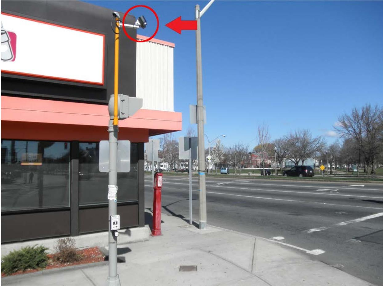
**Figure 23. Photo. Operational stereo pedestrian detection system on the south side of Broadway and the west side of McGrath Highway in Somerville, MA.**
