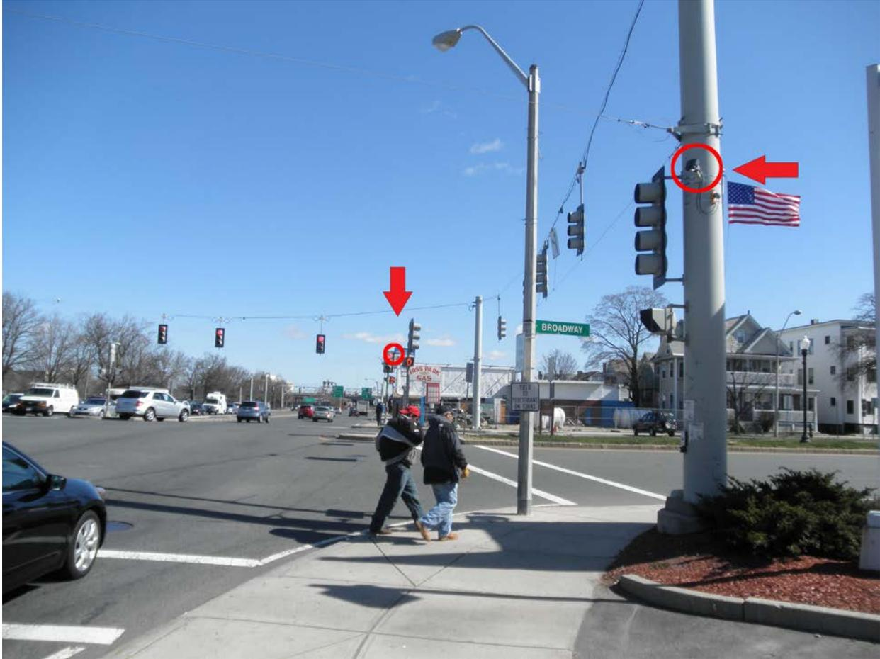
**Figure 20. Photo. Operational stereo pedestrian detection system at the intersection of McGrath Highway and Broadway in Somerville, MA.**
