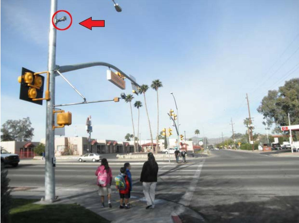
**Figure 18. Photo. Operational stereo pedestrian detection system at the intersection of West Kelso Street and North Oracle Road in Tucson, AZ.**
