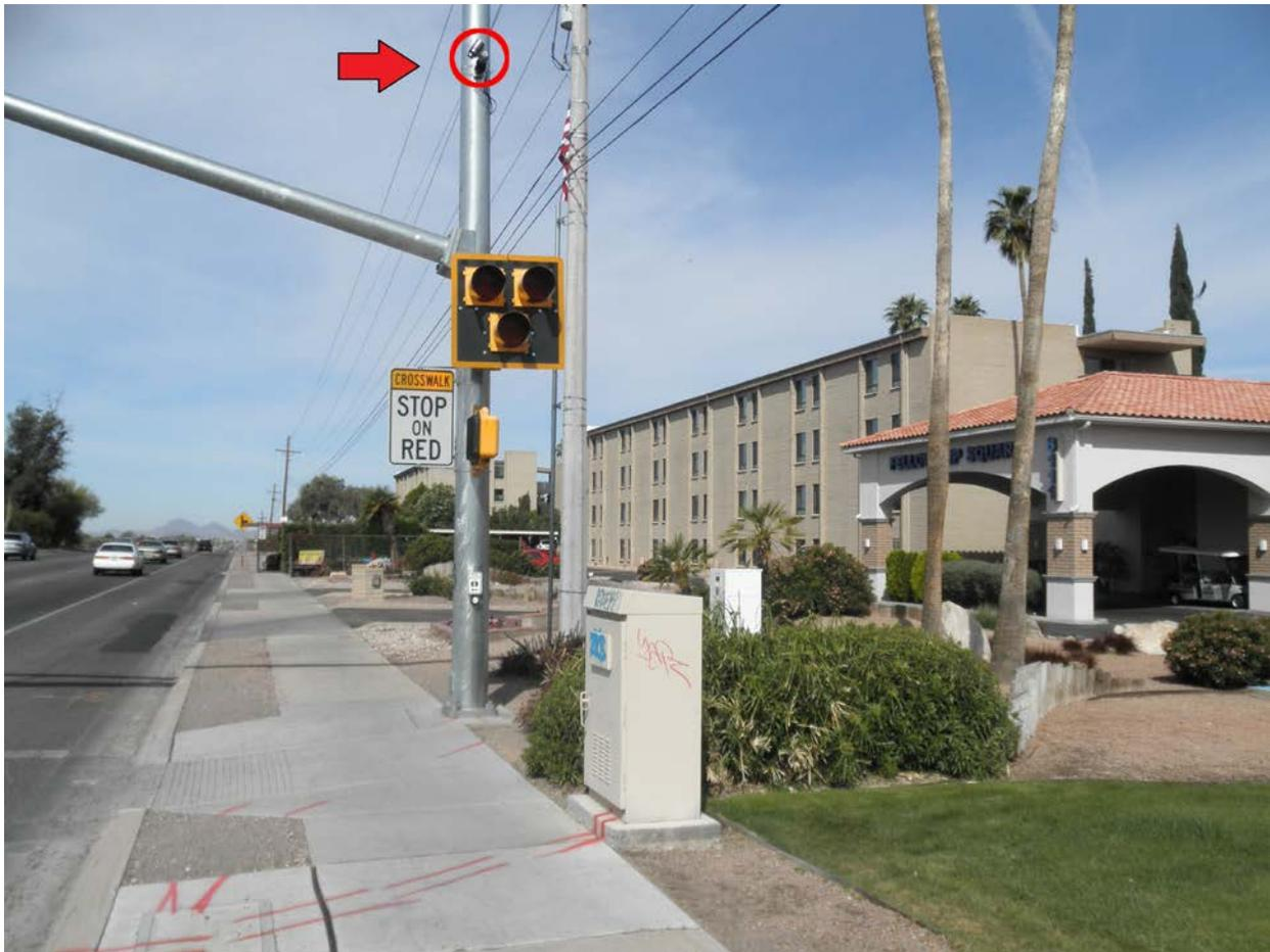
**Figure 16. Photo. Operational stereo pedestrian detection system on East Broadway at Fellowship Square in Tucson, AZ.**
