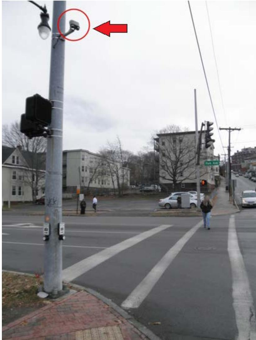
**Figure 24. Photo. Operational stereo pedestrian detection system on the northeast corner of Deering Avenue and Park Avenue in Portland, ME.**
