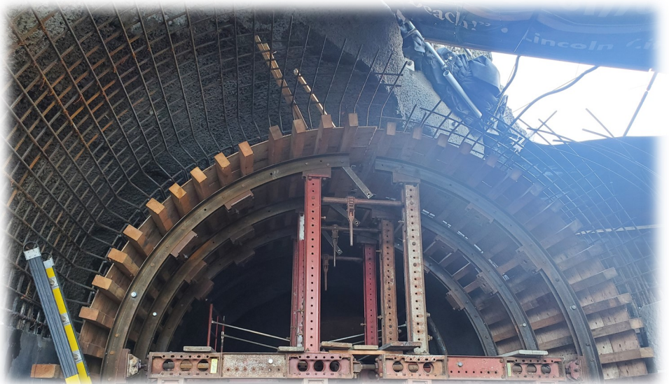
All forming the next arch section at the East Portal
