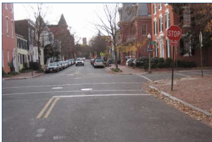
Double-yellow centerline and stop bars added to existing (24-inch) stop sign.
