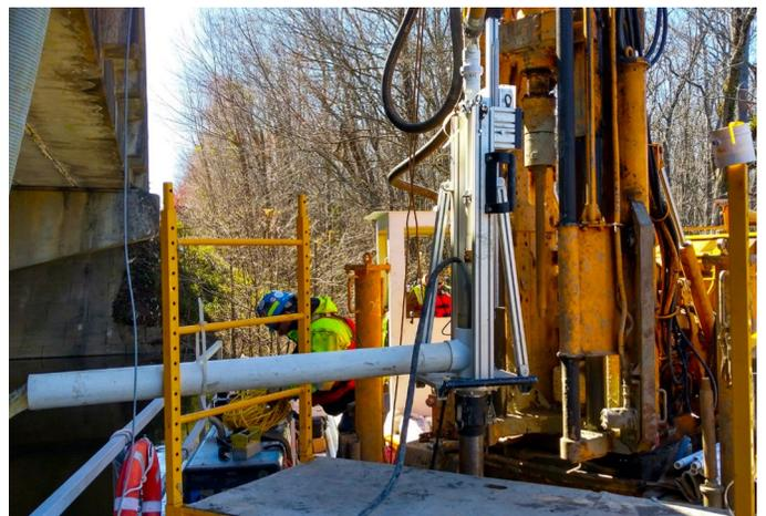
The ISTD equipment assembled in front of the drill rig on the barge.
