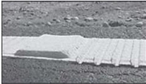
Figure 2. Photo. Inverted profiled thermoplastic marking.<sup>(1)</sup>
