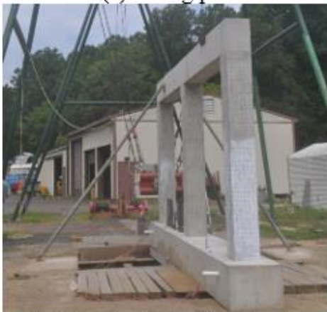
(c) Back view of the pier-bent.
