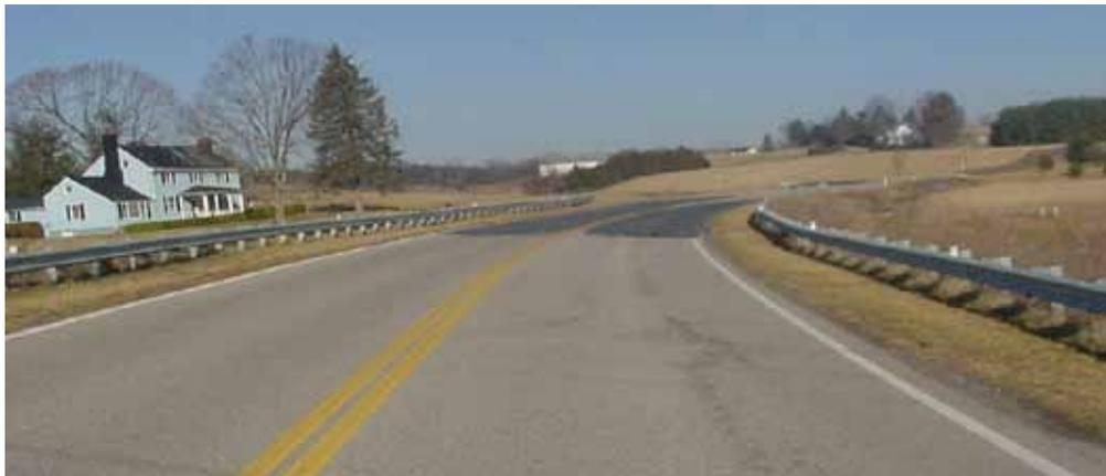
**Figure 20. Example bituminous surface treatment.**
