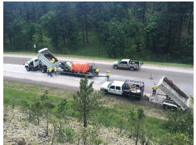
Figure 3: Semi-Automated HFST Application Method. Source: SDDOT
