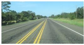
Center line buffer area at TX-21. Source: TTI
