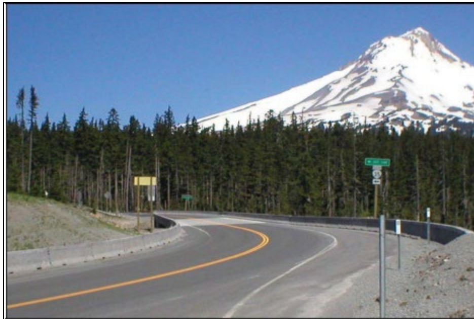
Figure 66. Photograph. Example concrete safety shape. (59)
