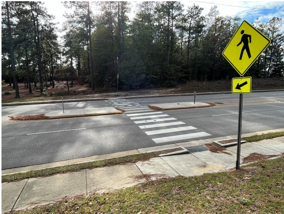
Figure 52. Photograph. Examples of non-motorist refuge.
