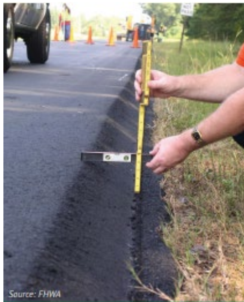
Figure 78. Photograph. SafetyEdge SM example. (68)
