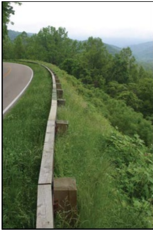
Figure 69. Photograph. Example steel-backed timber rail. (59)
