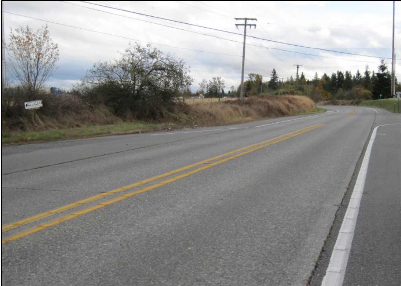
Figure 82. Photograph. Example of profile thermoplastic pavement markings. (66)
