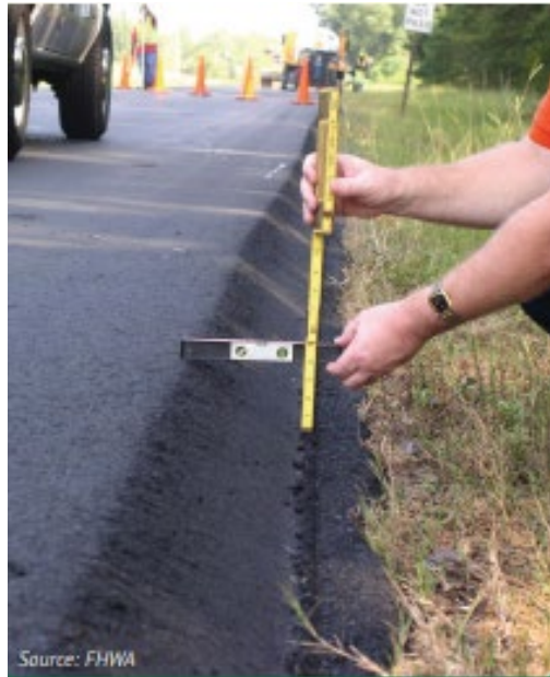
Figure 109. Photograph. SafetyEdge SM example. (68)
