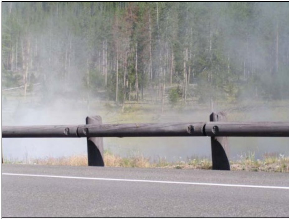
Figure 106. Photograph. Example steel-backed log rail. (59)
