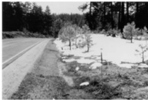
Typical Roadway with Roadside Hazard Rating Equal to 3.
