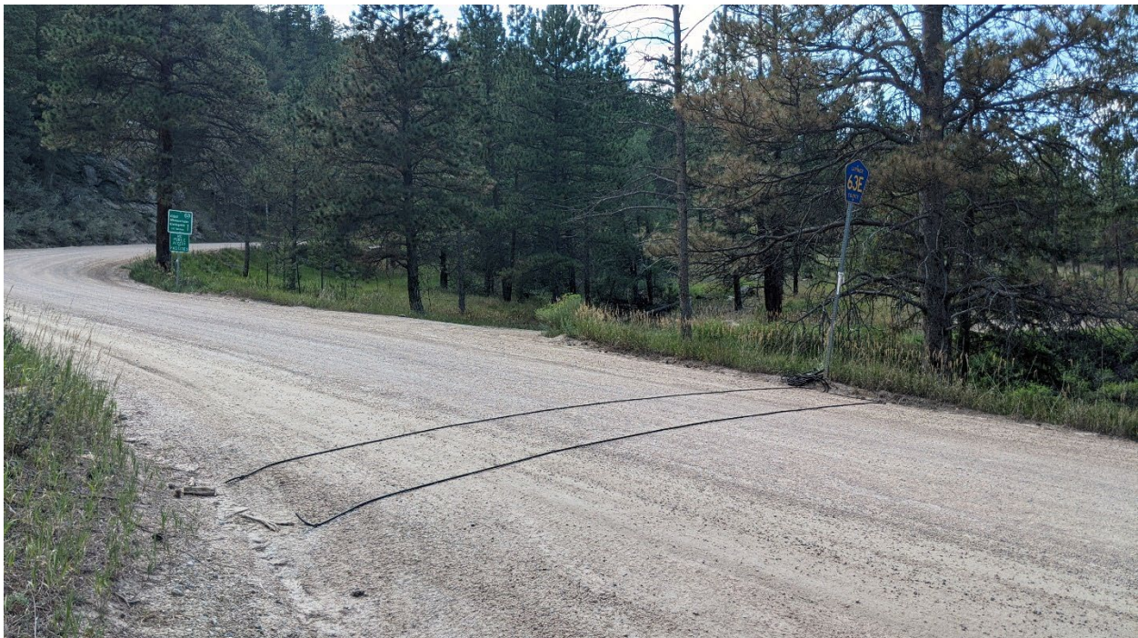
Figure 41. Photograph. Example of an active traffic count in progress.
