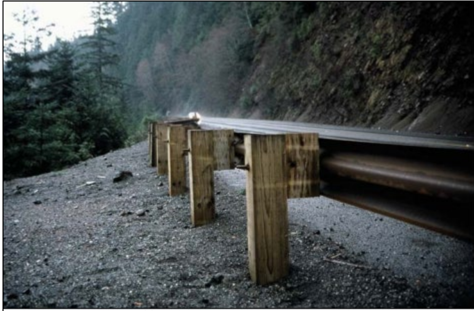
Figure 71. Photograph. Example strong post w-beam. (59)
