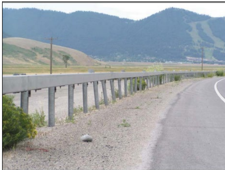
Figure 70. Photograph. Example box beam. (59)
