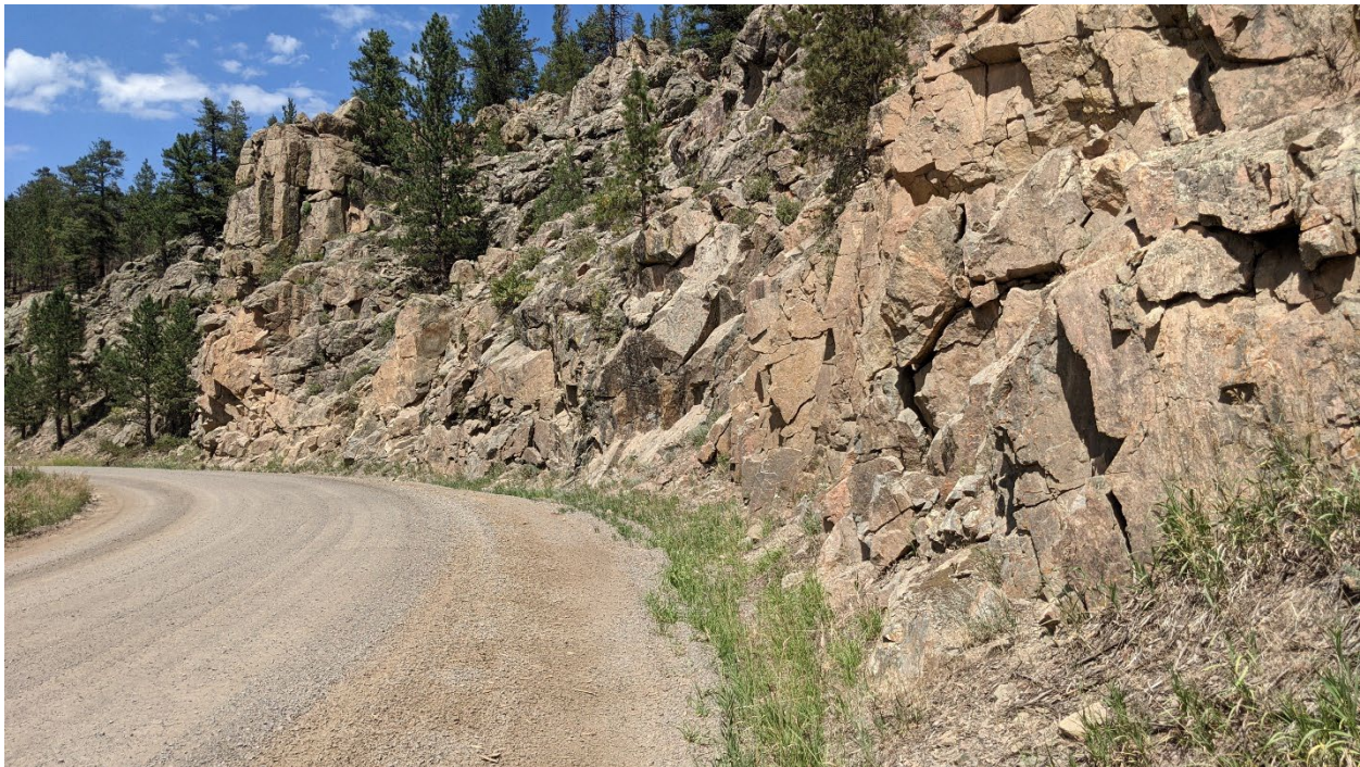
Figure 55. Photograph. Example of a narrow recoverable area.
