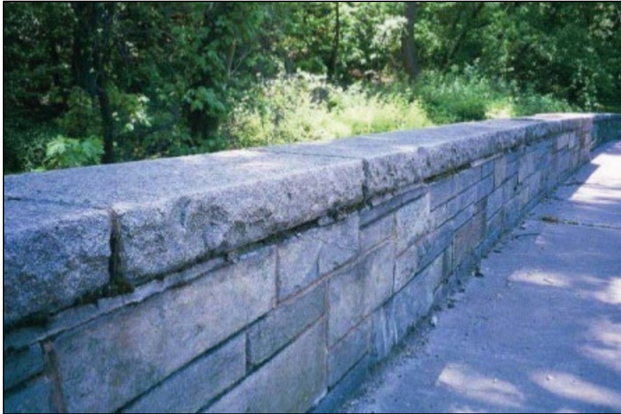
Figure 67. Photograph. Example precast concrete guardwall. (59)
