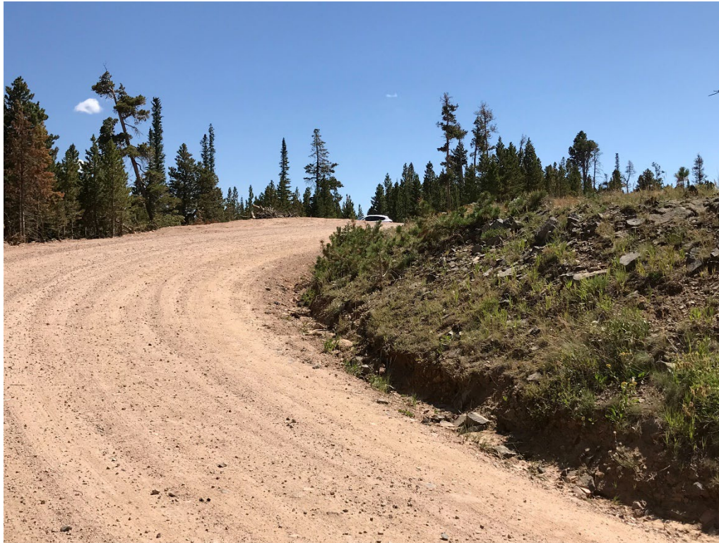
Figure 43. Photograph. Break in the tree line providing a visual cue that can be a potential visual trap.
