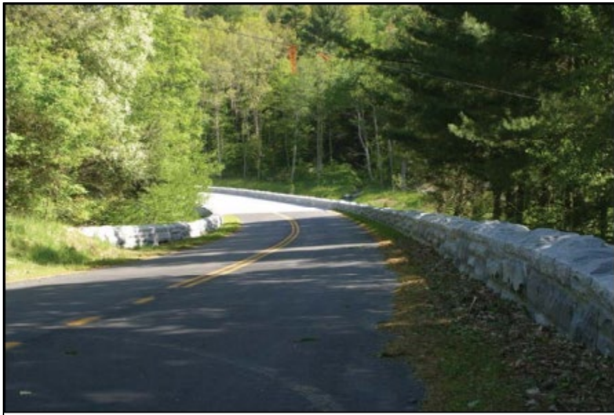
Figure 67. Photograph. Example precast concrete guardwall. (59)
