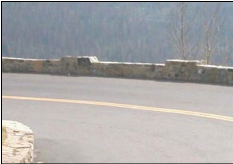
Figure 77. Photograph. Example random rubble cavity wall. (59)
