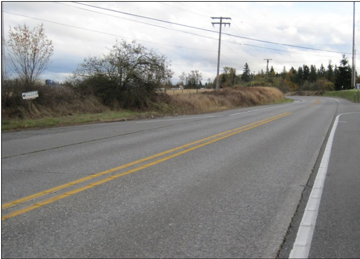
Figure 64. Photograph. Example of profile thermoplastic pavement markings. (66)
