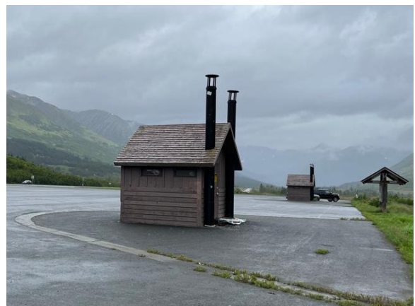
Image 4 Existing Bathroom Facilities at Moto Lot
