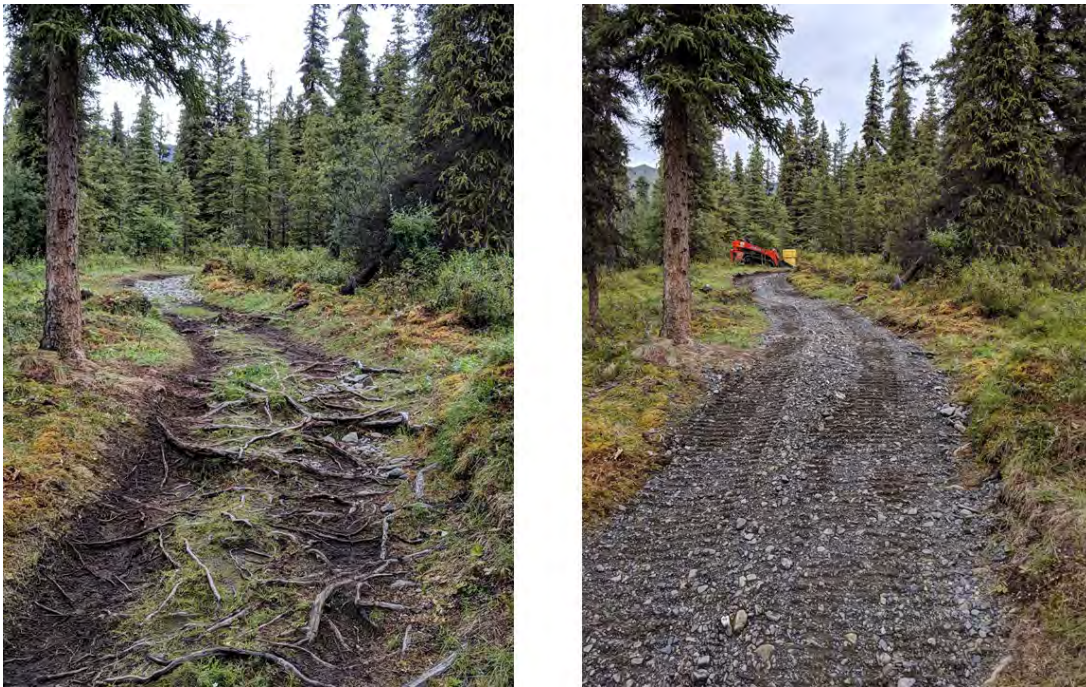
Figure 5: Gravel Use in Trail Construction for Caribou Creek Trail before (left) and after (right). Source: NPS
