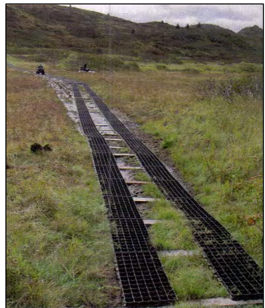
Figure 7: Example of a “GeoTrack” used in trail maintenance on Kodiak Island. Source: GeoChem, Inc.
