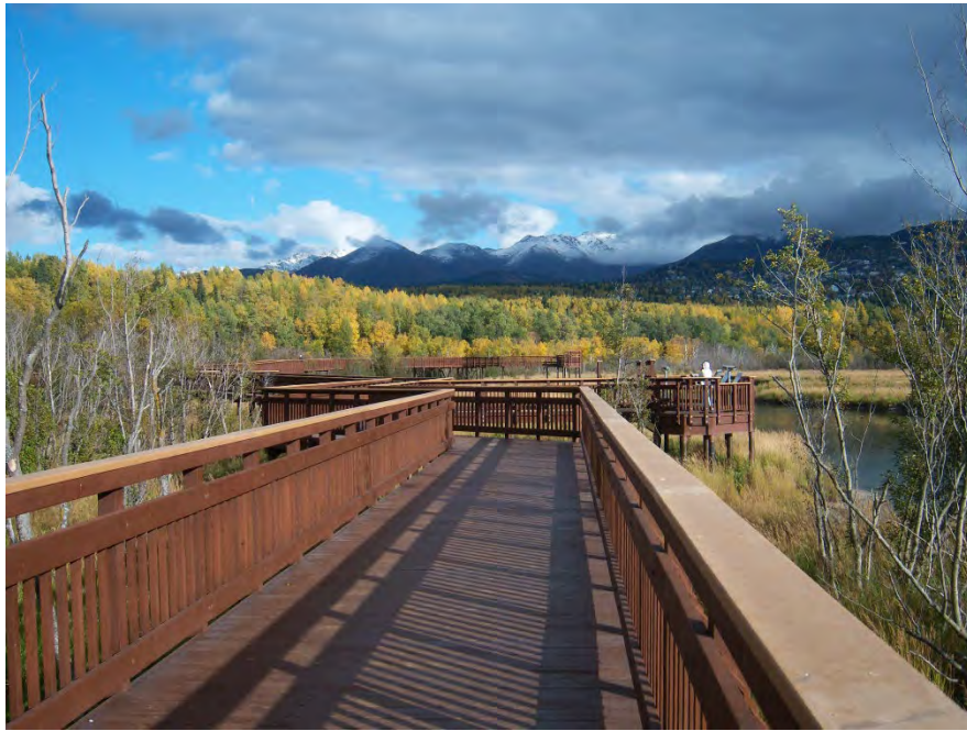
Figure 10: Elevated trail on helical piles from Potter's Marsh, Anchorage Coastal Wildlife Refuge . (Source: NPS)
