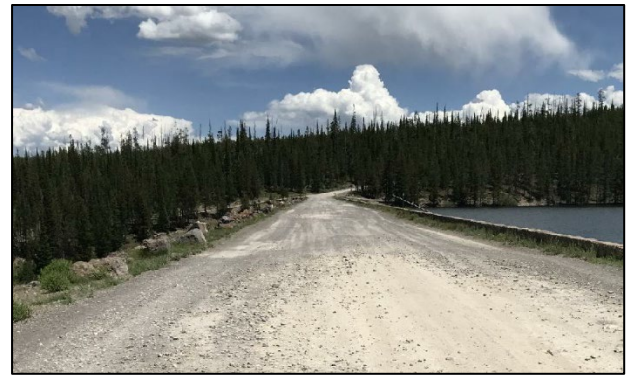
Figure 13: AFRR at Grassy Lake Reservoir (MP 22.5)
