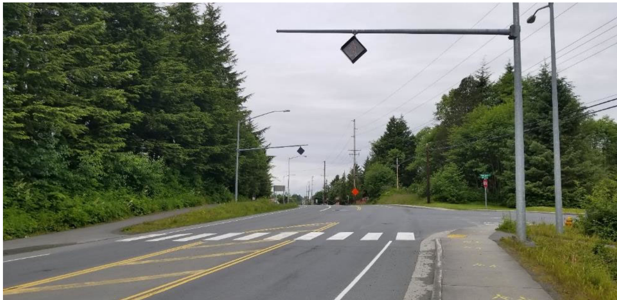
Figure 7 - A lighted sign hangs above a crosswalk at the intersection of Indian River Road and Sawmill Creek Road.
