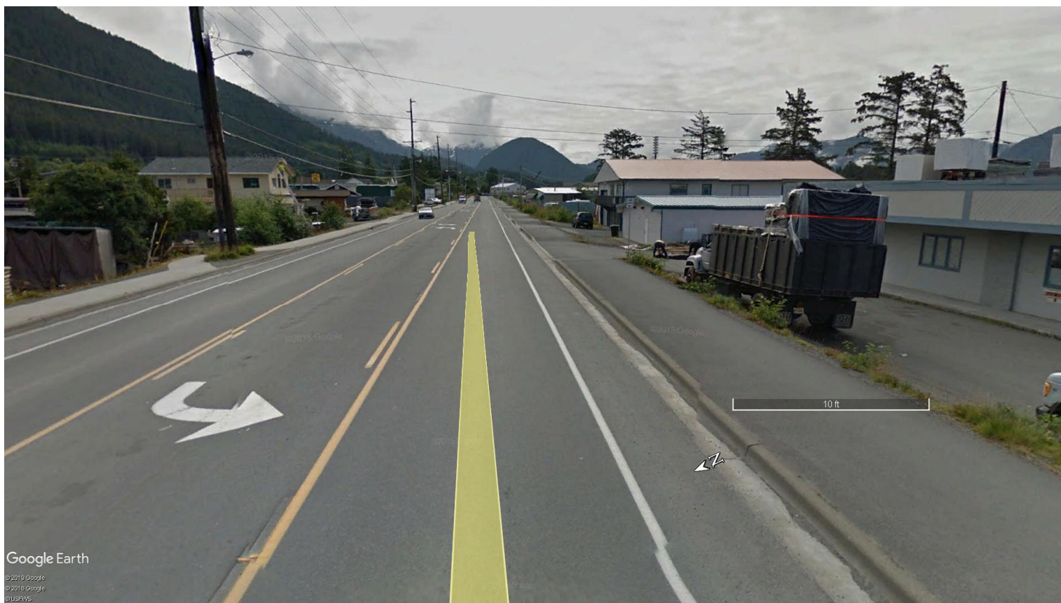
Figure 38 - Existing Shared-Use Path Along SMC Road East of Study Area, Approx. 10' Wide
