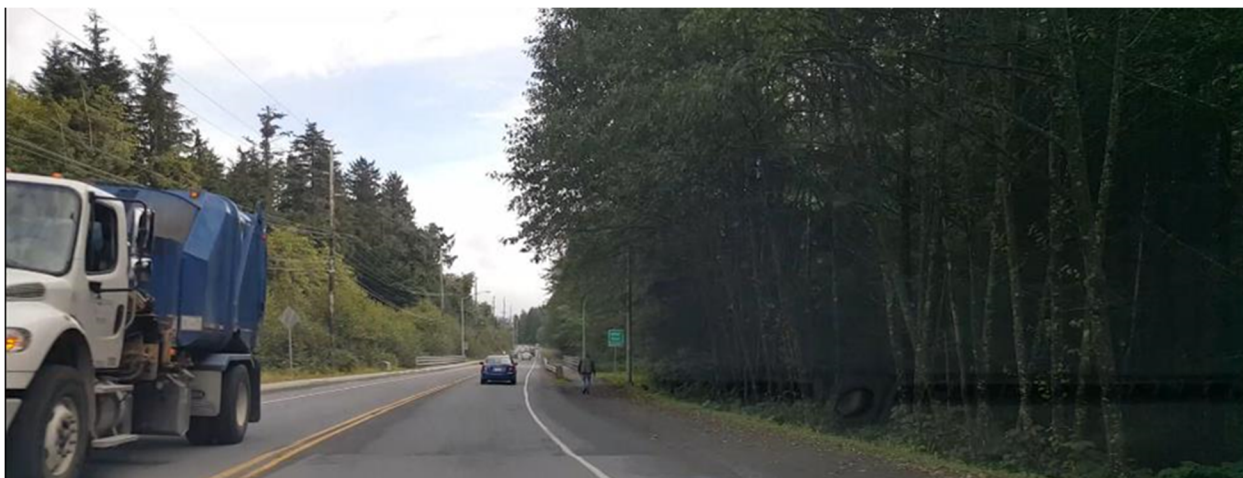
Figure 25 - EB Sawmill Creek Road approaching Indian River Bridge
