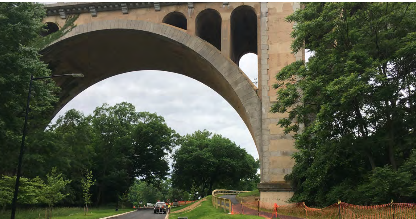
View of the Connecticut Avenue NW bridge from Beach Drive
