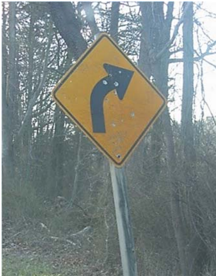
Patuxent Research Refuge non-compliant signage observed during a Road Safety Audit. Photo by VHB
