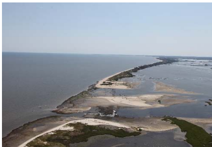
Breach at Prime Hook NWR following Hurricane Sandy. Photo by FWS
