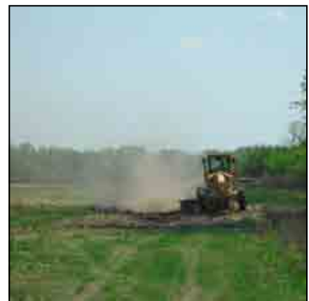
Road construction at Flint Hills NWR.
