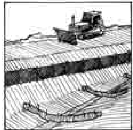
Standard practices such as using silt fencing help reduce construction impacts to adjacent habitat.
