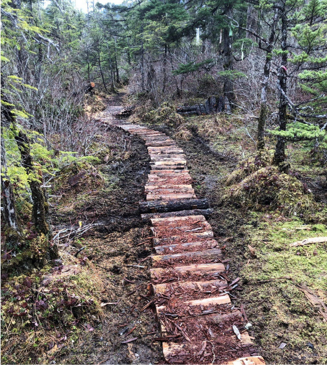
Figure 6. Makeshift boardwalk created with logs through sensitive muskeg habitat along the Bonnie Brae access trail.
