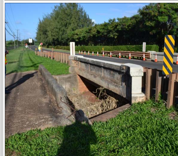
Hoolapa Bridge, Pre-Construction
