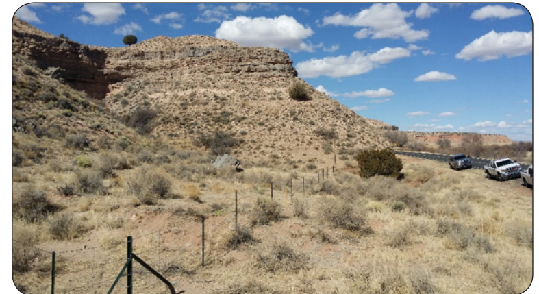
Fencing installed in hilly area near Sunrise, Arizona
