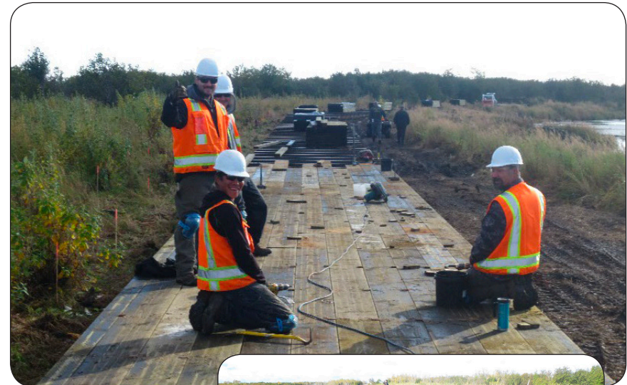
Crew installing boards onto the steel framing.
