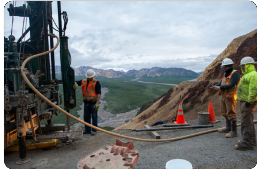
Drilling on Denali Park Road in the middle of the Pretty Rocks Landslide with the Alaska Range visible in the background.
