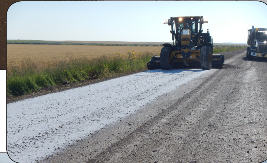
Application of \text{CaCl}_2 , Malmstrom Air Force Base, Montana
