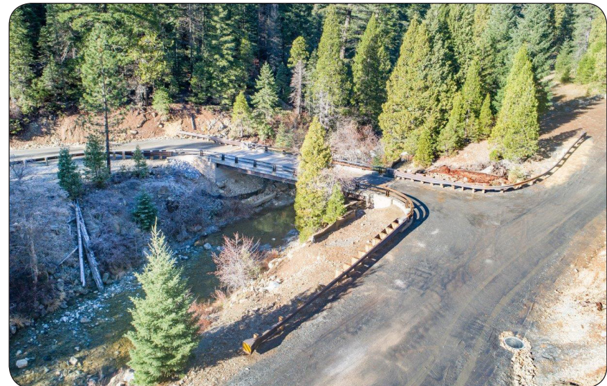
Mumbo Creek Bridge, California
