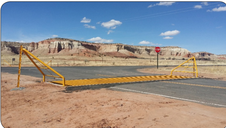
Fencing and cattleguard installed at Cornfields Chapter Access Road, Arizona
