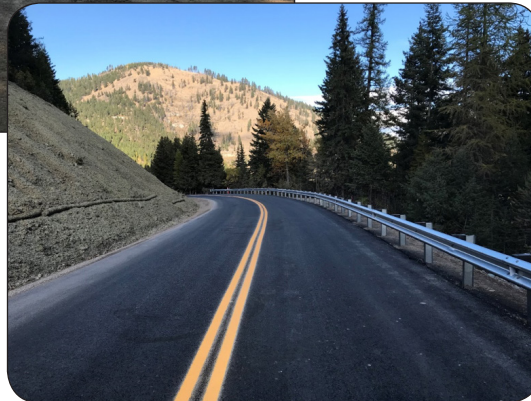
The completed project.
