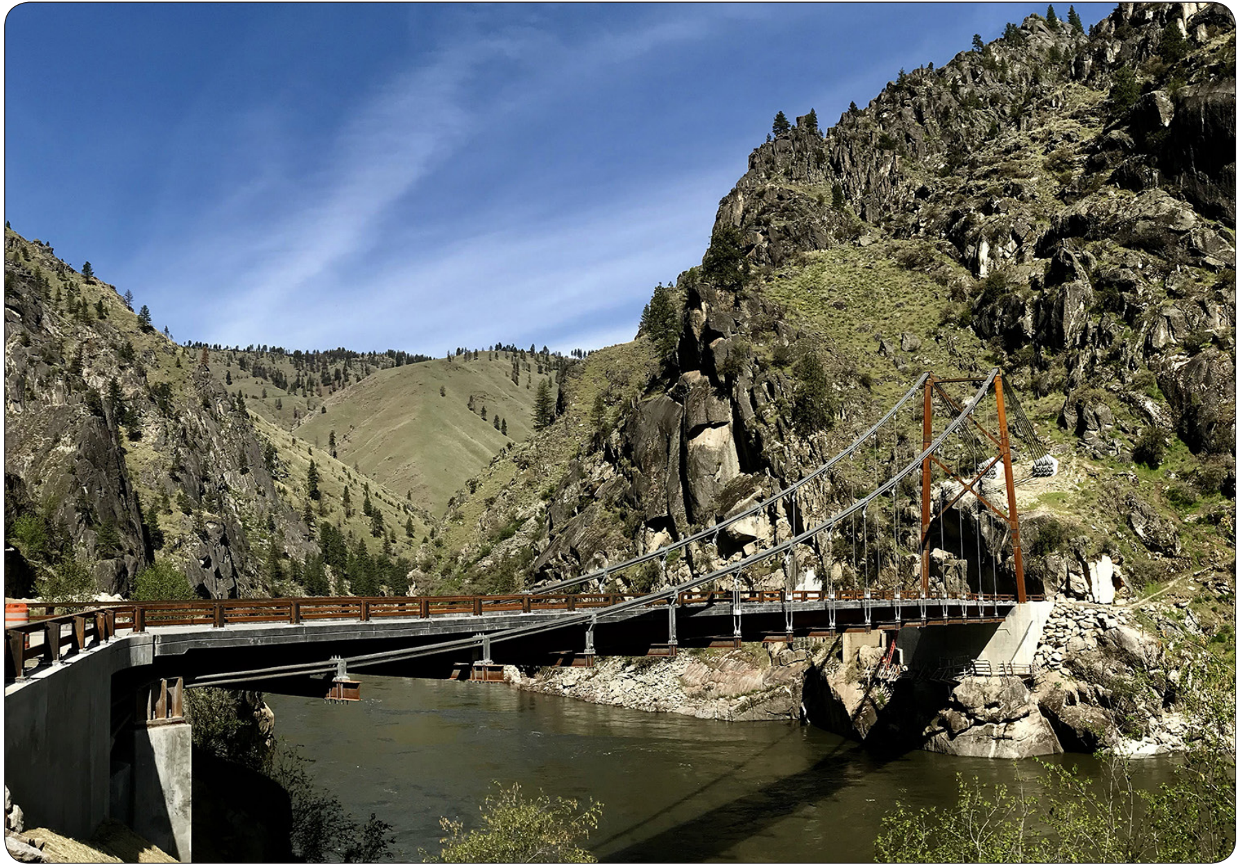
Manning Crevice Bridge, Salmon River Road, Idaho
