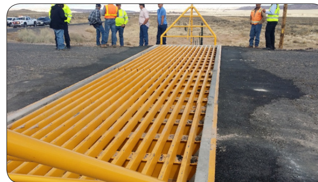
Three Unit Cattleguard Installation at Greasewood Springs Access Road, Arizona
