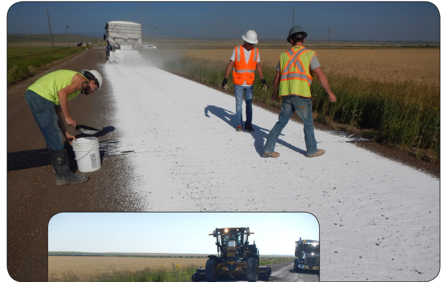
Application of \text{CaCl}_2 , Malmstrom Air Force Base, Montana
