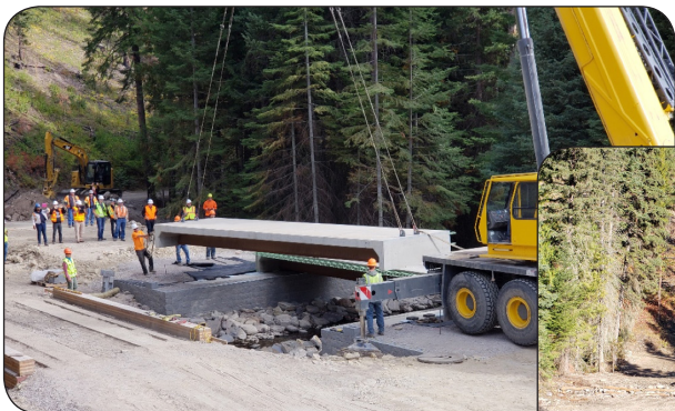
North Valley Creek Bridge Replacement, Flathead Indian Reservation, Montana Located northwest of Arlee, Montana on the Flathead Indian Reservation, this project removed an existing timber bridge over North Valley Creek and constructed a new 35-foot folded plate girder bridge with GRS abutments and superstructure. Construction and Construction Administration was managed by the Confederated Salish and Kootenai Tribes force account using Confederated Salish and Kootenai Tribes' TTP funds and an Accelerated Innovation Deployment Grant.
