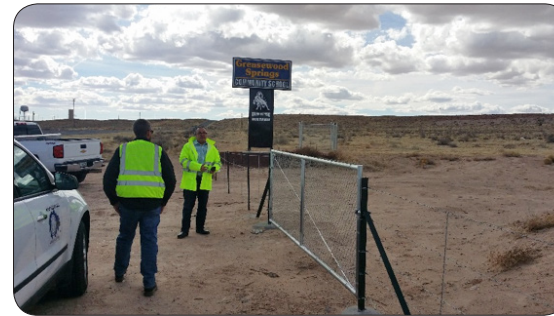
Gate installation for Access to Greasewood Springs School, Arizona
