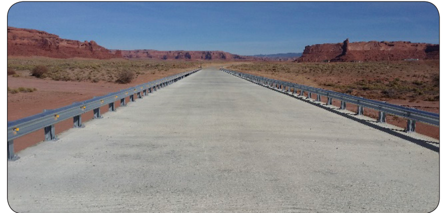
Looking east along concrete deck of new bridge.
