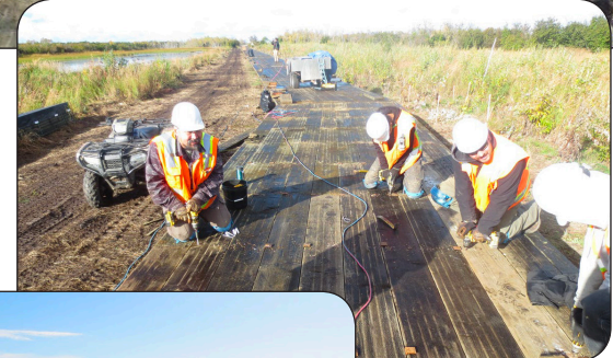
Crew installing boards onto the steel framing.
