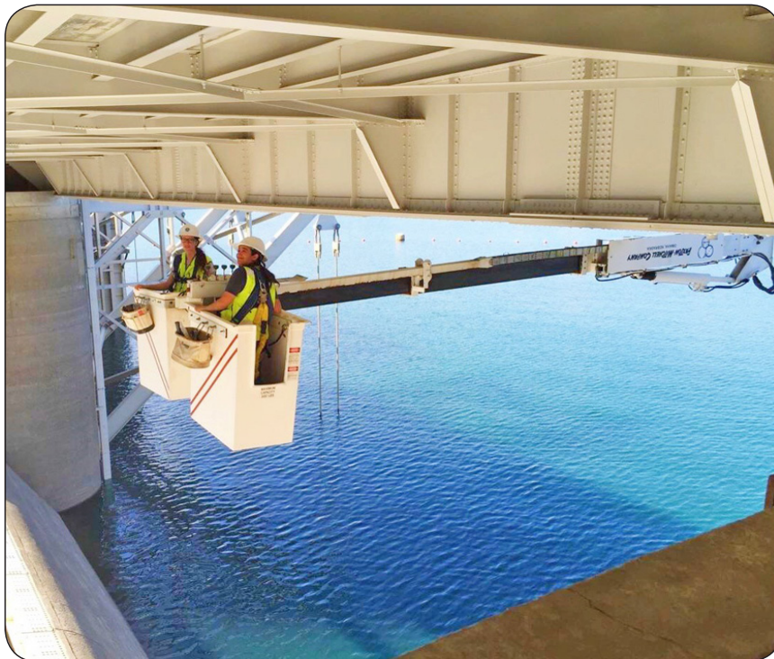
Under Bridge Inspection, Lake Shasta Spillway Bridge, California
