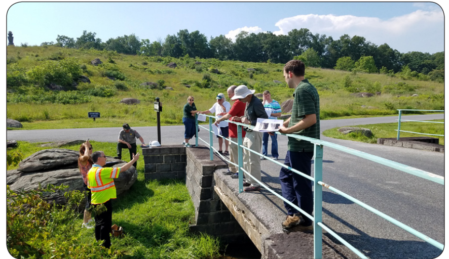
FLH Bridge Management Team reviewing process for bridge inspections with NPS staff during the annual Roads Working Group meeting, Gettysburg, PA
