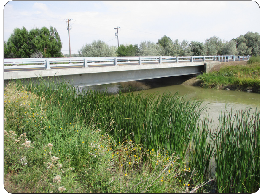
Old Highway 2 Rehabilitation and Bridge Replacement, Phillips County, Montana
