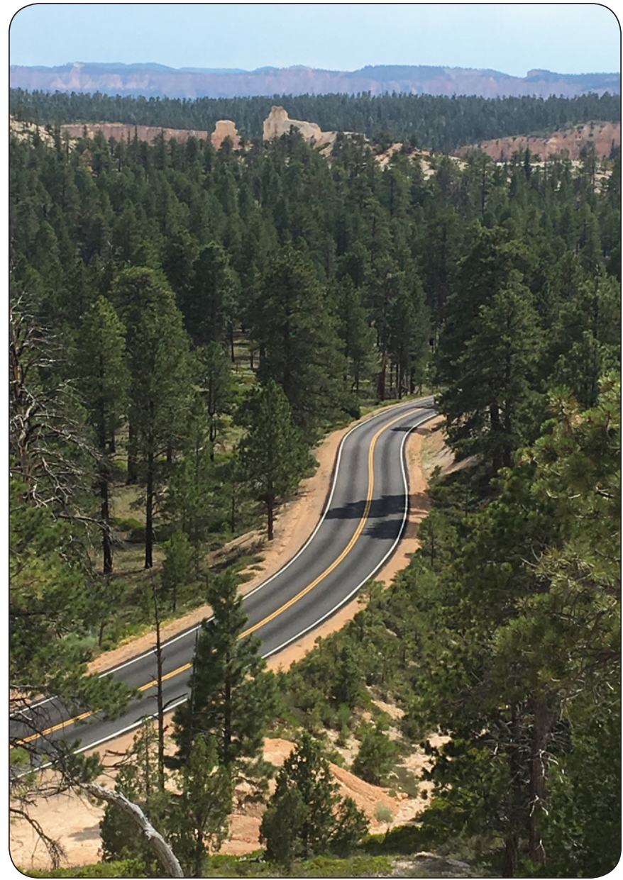
Bryce Point Access Road, Bryce Canyon National Park, Utah
