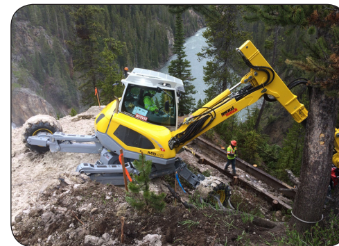
Boardwalk Installation at Inspiration Point, a viewpoint on the north rim of the Grand Canyon of the Yellowstone River, Yellowstone National Park, Wyoming
