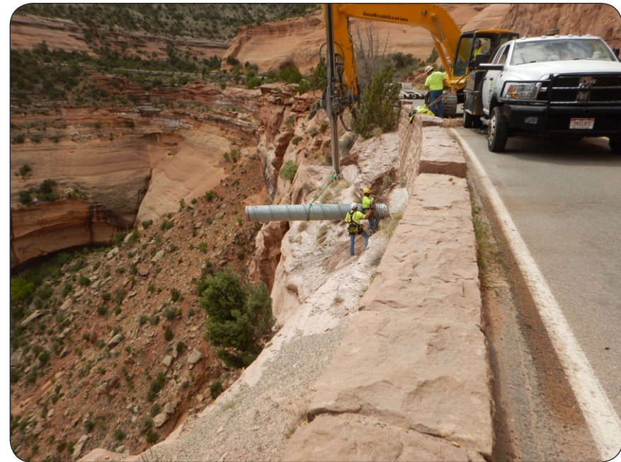
Culvert Installation, Rim Rock Drive, Colorado National Monument, Colorado
