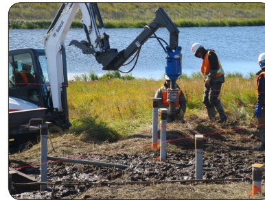
Installation of helical piers
