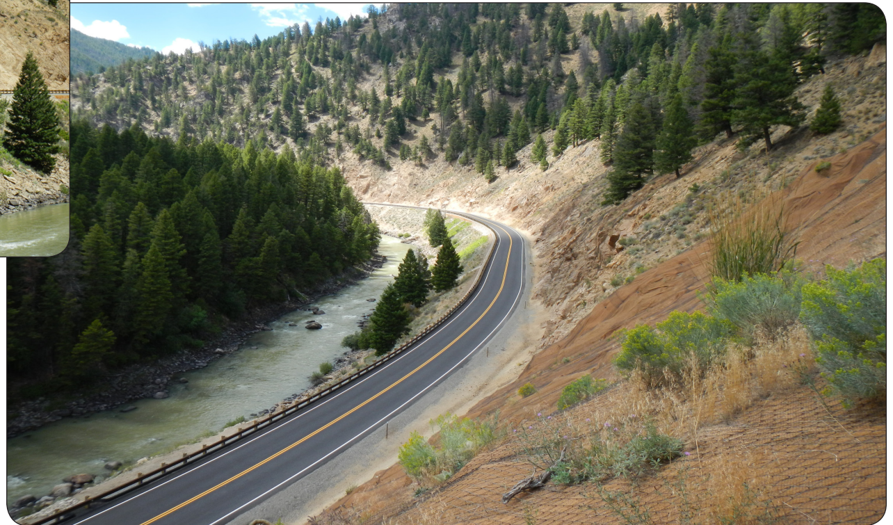
Contoured mesh and rock pins barely visible on the slopes
