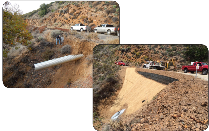
Drainage Repairs (Before & After), Figueroa Road, Los Padres National Forest, California
