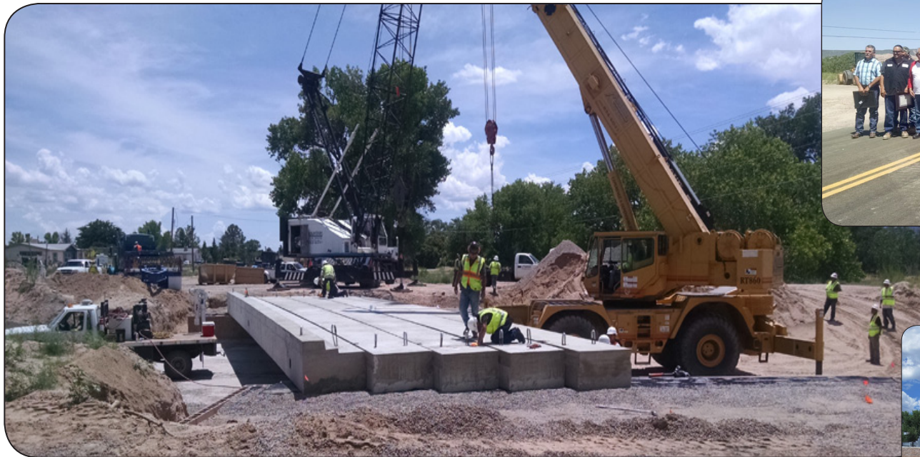
Setting last girder into place and view of completed bridge
