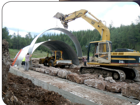
FLAP road reconstruction and installation of Aquatic Organism Passage and Animal Crossings, New Mexico State Highway 126, Jemez Mountain Trail National Scenic Byway, New Mexico
