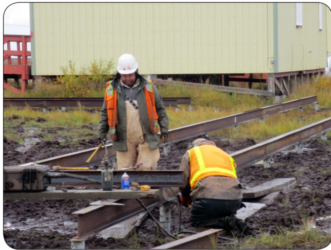
Welding and assembly of boardroad framing
