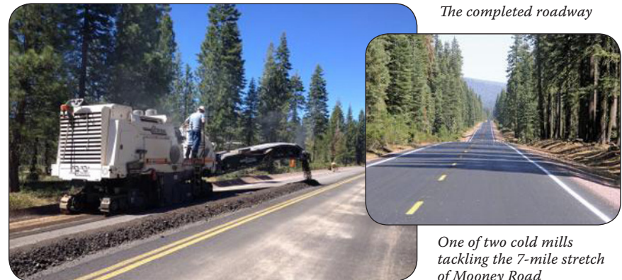
The completed roadway
