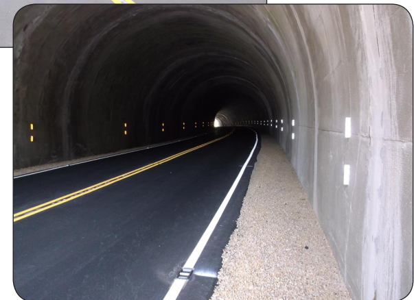
Devil's Courthouse Tunnel stone portal entrance and inside look at the new concrete lining
