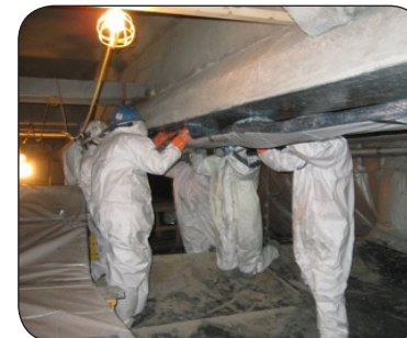
Carbon Fiber Wrap being installed after repair of beam surface
