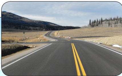
Completed roadway view looking north of the Sevenmile Valley
