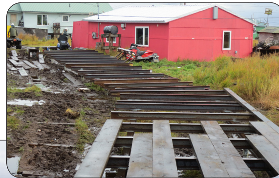
Board installation on steel framing
