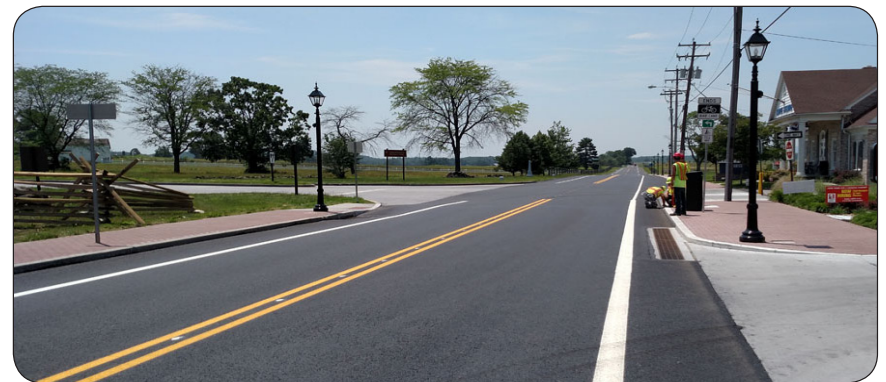
Looking south toward Park Entrance (on left) note drainage improvements
