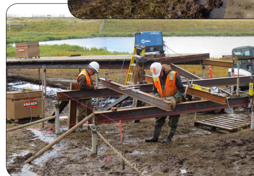
Framing in preparation for welding
