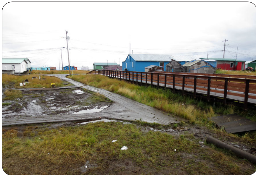
Old Boardroad adjacent to the new replacement
