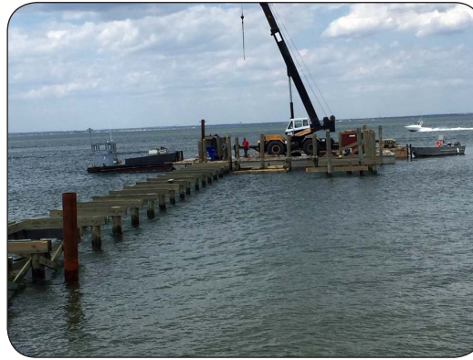
Pile driving from construction barge
