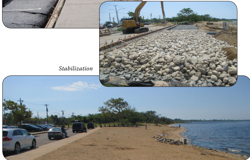
View of the completed project
