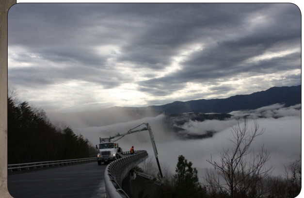
Under Bridge Inspection Vehicle (UBIV), Foothills Parkway, Tennessee
