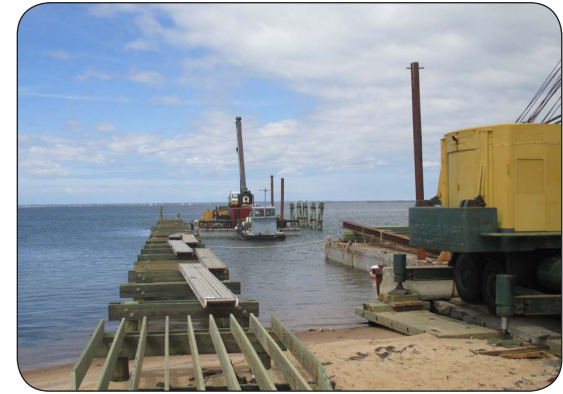
Reconstructing water taxi dock
