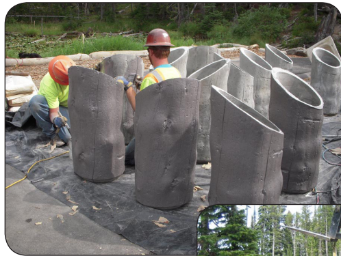
Painting the concrete (simulated wood) pier caps
