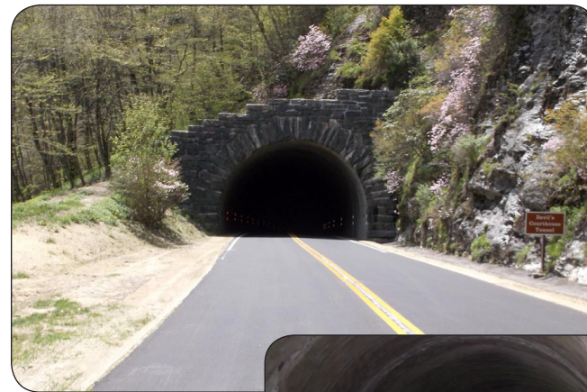
Devil's Courthouse Tunnel stone portal entrance and inside look at the new concrete lining
