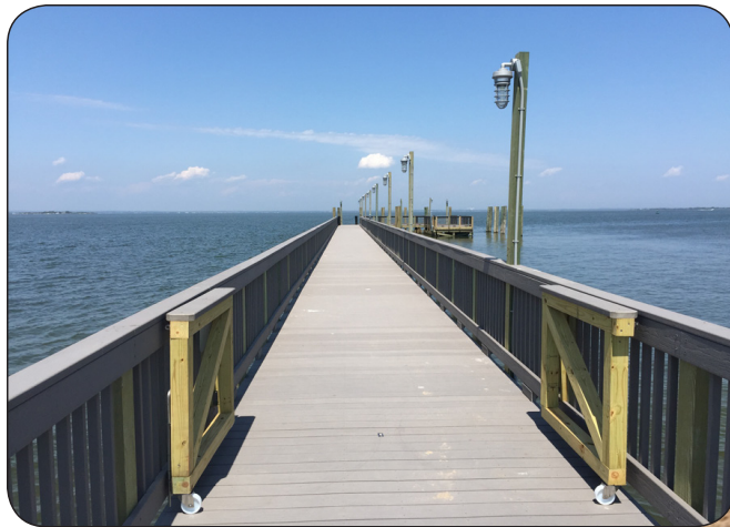
Views of the completed dock
