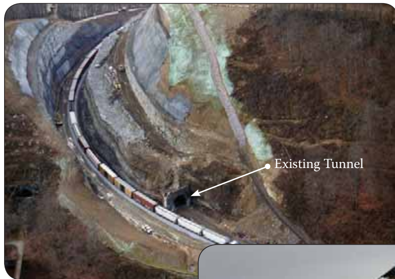
Train traffic continues to travel through the Pinkerton Tunnel Run-Around-Track while construction is underway to remove the existing tunnel. — Markelton, Pennsylvania
