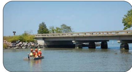
Under Bridge inspection via waterway, Colonial Parkway, VA
