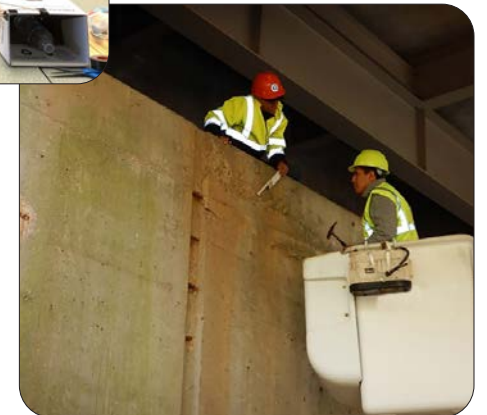
Bridge Inspection Field Trip, Turkey Run Bridge, George Washington Memorial Parkway, Virginia
