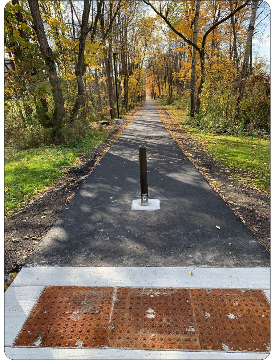
Penny Trail, a newly revitalized multi-use trail project, was completely administered by the Seneca Nation through a 202(a)(9) agreement. A former railroad route on the Western New York and Pennsylvania Railroad System, the trail was widened and paved to include safety enhancements with installation of lighting, bollards, signage and emergency call boxes. Salamanca, New York
