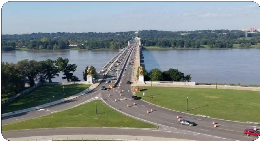
Arlington Memorial Bridge Rehabilitation completion of Phase 1, Washington DC/Arlington, Virginia
