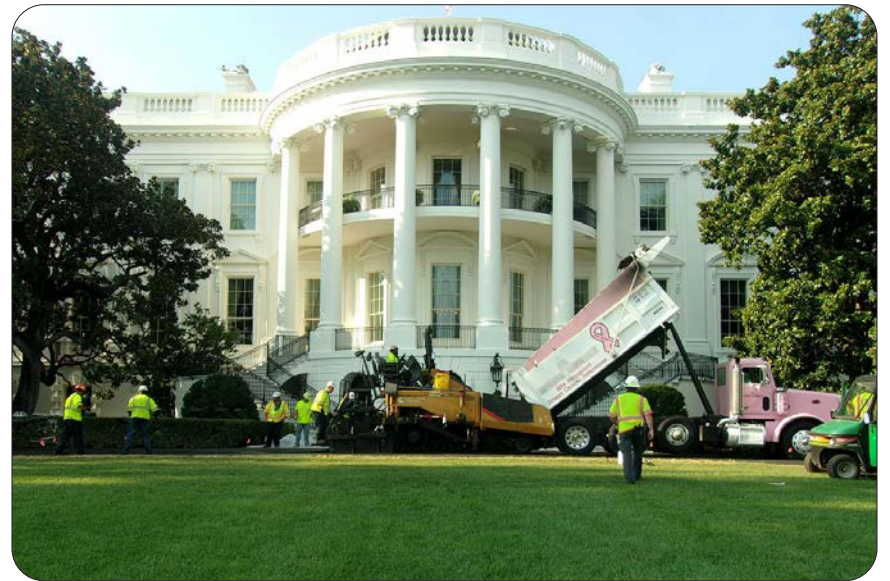
President's Park and White House pavement resurfacing work and full depth pavement patching completed on Ellipse Road, South Grounds Road, and associated connection roads. Washington, DC
