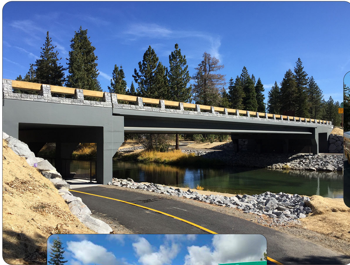
Truckee River Bridge, Tahoe City, California
