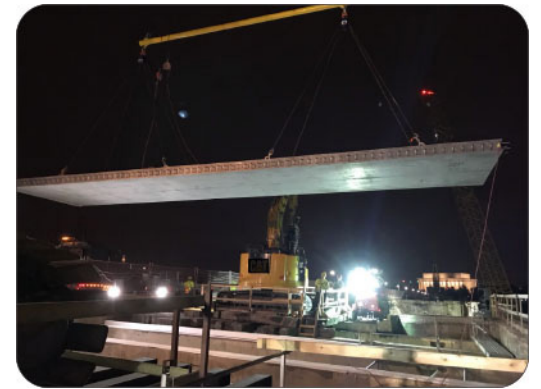
Precast concrete deck installation
