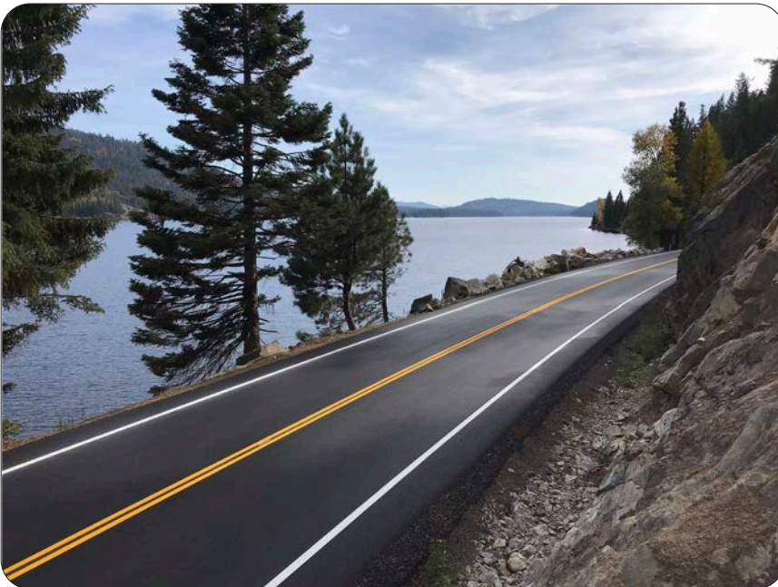
Views of Warren Wagon Road located along Payette Lake and the North Fork Payette River was reconstructed with frost-resistant pavement improving safety and drainage while minimizing future maintenance. Valley County, Idaho
