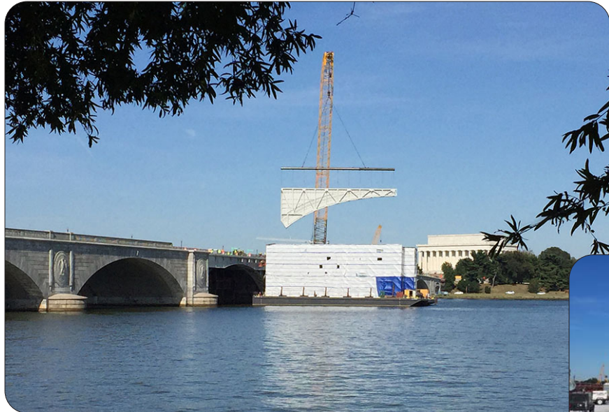
Installation of restored drawbridge face maintains the historic character of the bridge, Arlington Memorial Bridge, Washington DC/Arlington, Virginia
