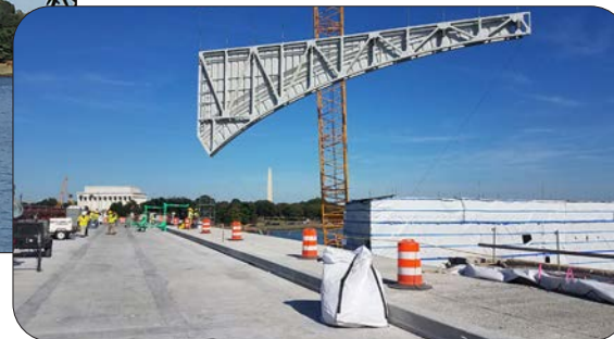
Installation of restored drawbridge face maintains the historic character of the bridge, Arlington Memorial Bridge, Washington DC/Arlington, Virginia
